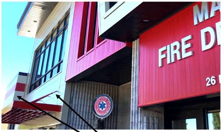
PROSED 12" WIDE METAL PANEL INSTALLED IN HORIZONTAL ORIENTATION
