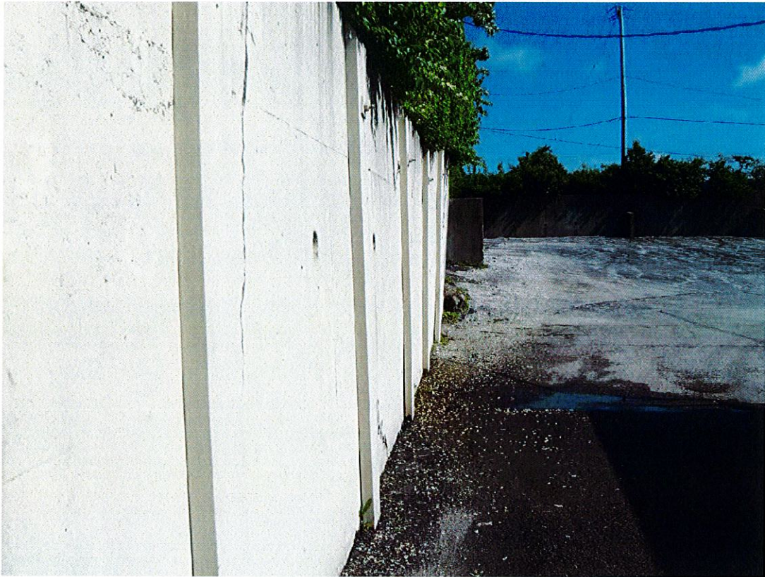
Photo 16 – Deteriorated/compromised retaining wall.
