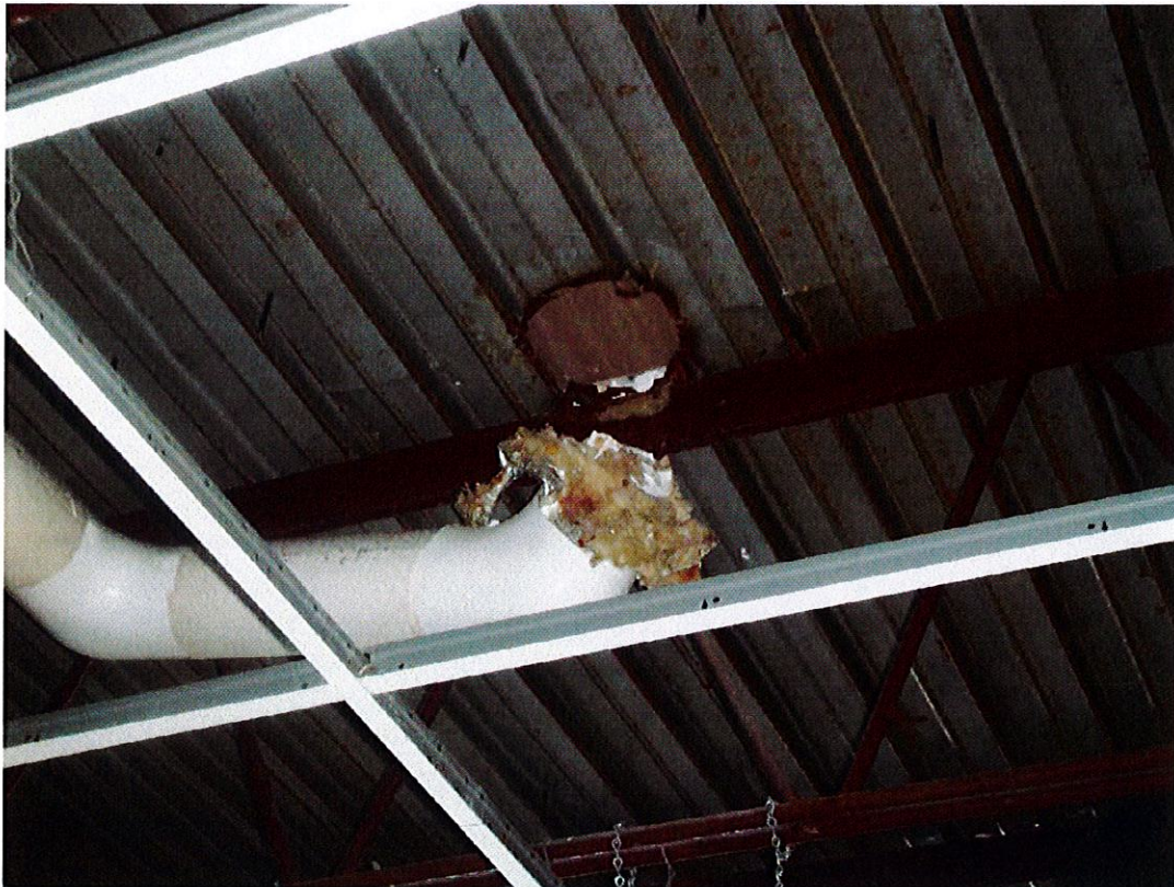
Photo 26 – Roof structure deterioration.
