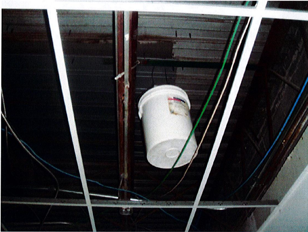
Photo 27 – Roof structure deterioration.
