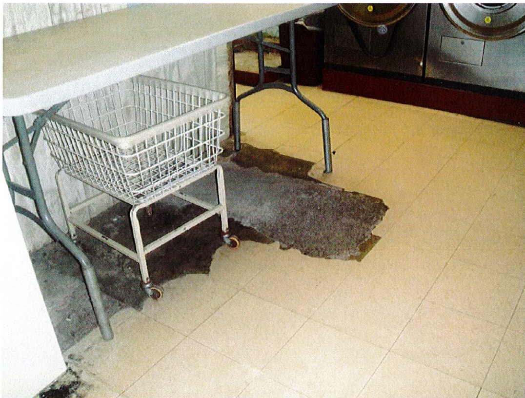
Photo 36 – Deteriorated/damaged floor tile.
