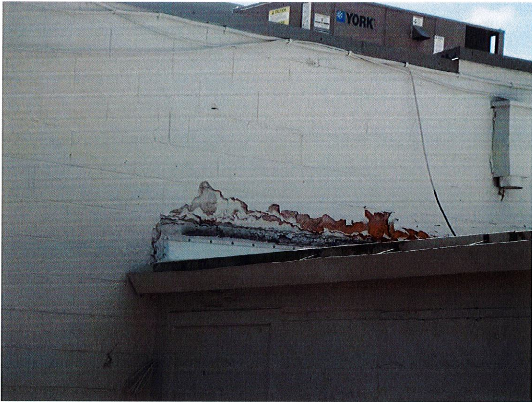
Photo 21 – Deteriorated flashing material.
