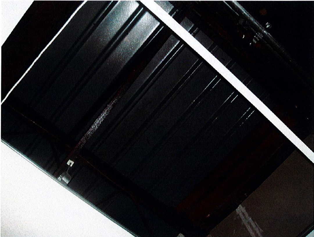
Photo 32 – Roof structure condensation.
