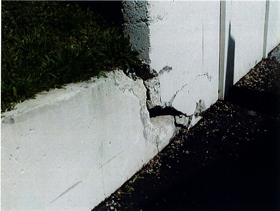
Photo 15 – Deteriorated/compromised retaining wall.
