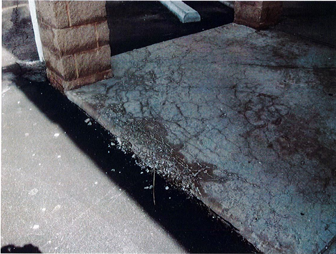
Photo 18 – Deteriorating concrete sidewalk.
