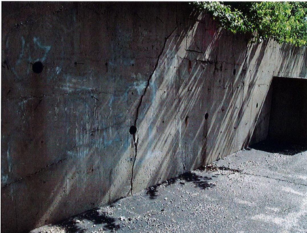
Photo 10 – Deteriorated/compromised retaining wall.
