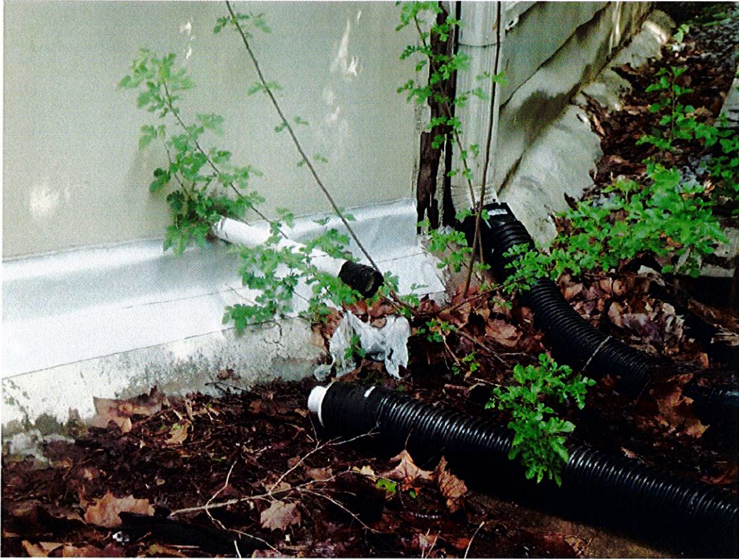
Photo 45 – Inadequate drainage area.
