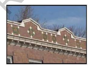
Parapet Wall Screening Roof Mounted Equipment
