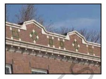
Figure 5.510.B-5: Parapet Wall Screening Roof Mounted Equipment
