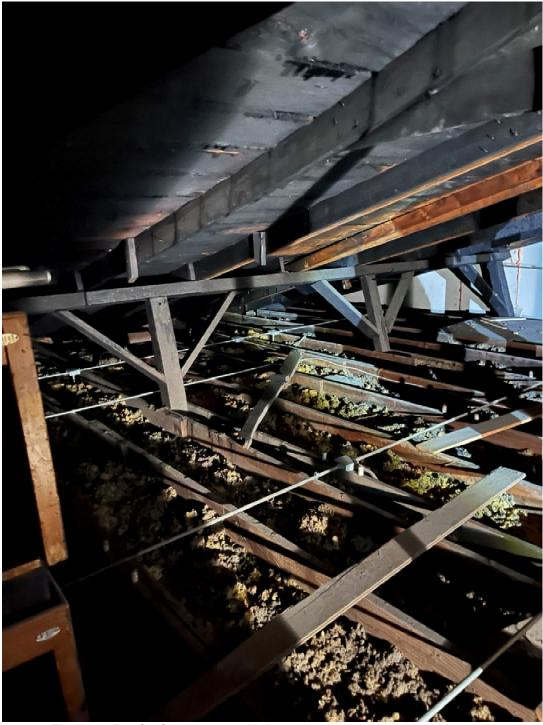
Figure 1. Roof rafter system with knee boards and tie rods.
