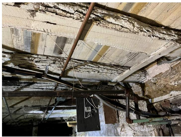
Figure 4. Rough lumber floor framing.
