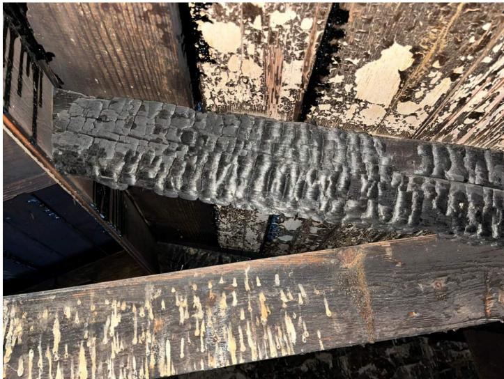
Figure 2. Fire damage of top chord of wood truss.
