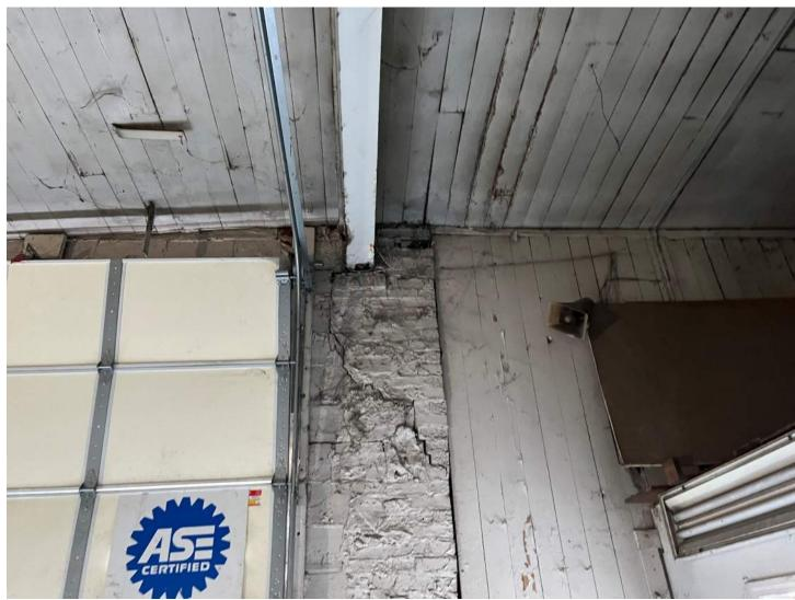
Figure 5. Settlement of stone exterior wall.
