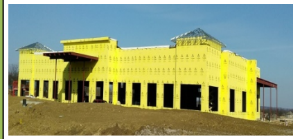
Control Service Company on Akin.
