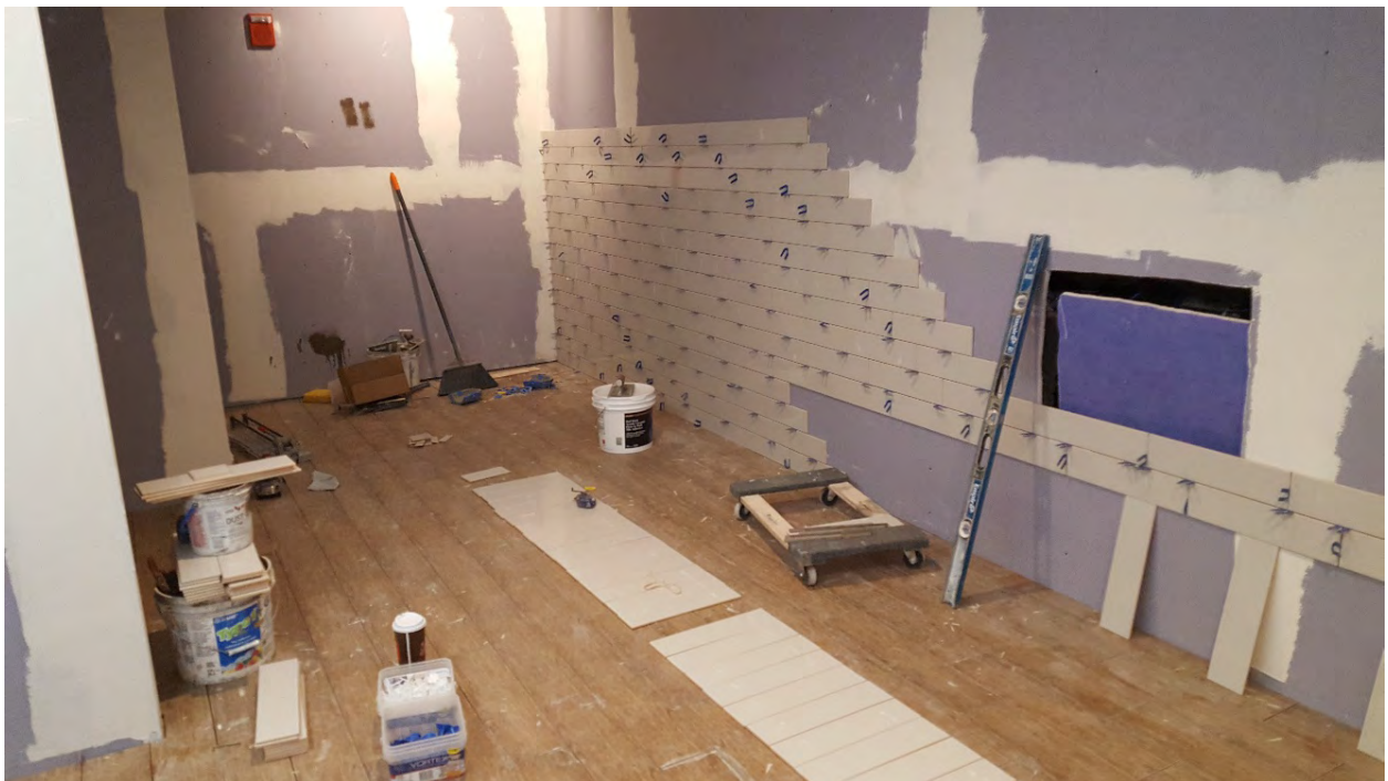
ABOVE: Floor and wall tile being installed in the men's restroom
