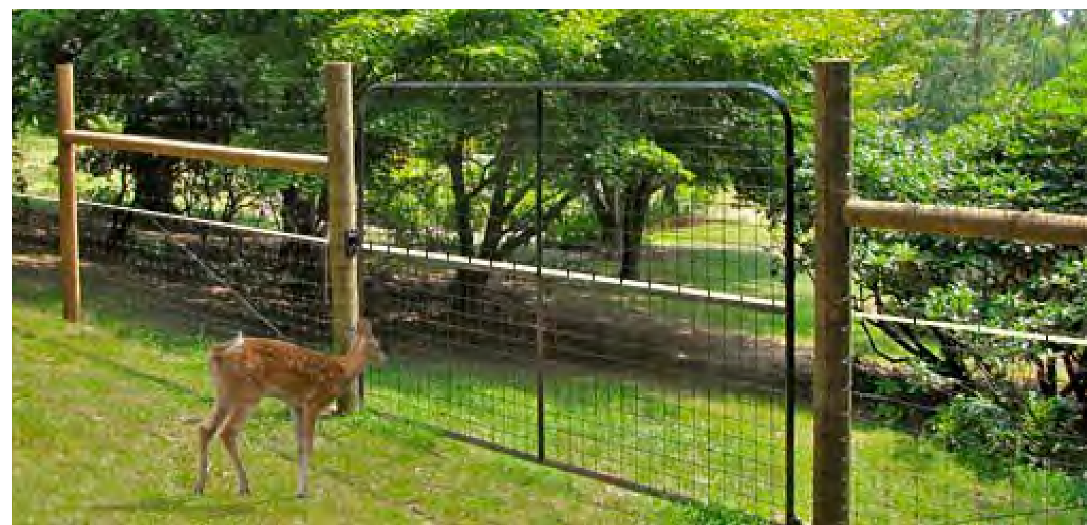
WILDLIFE FENCING: - More transparent means of restricting access to garden areas - Replaces existing chain link fence
