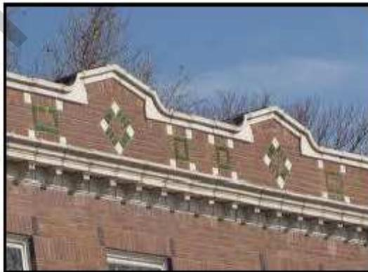
**Parapet Wall Screening Roof Mounted Equipment**
