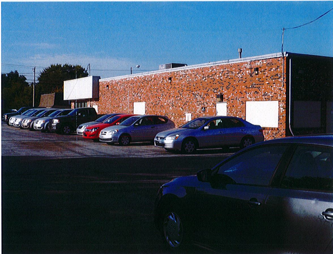
Looking southwest at 516 SW 3 rd Street
