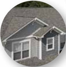
Roofing and Ventilation
