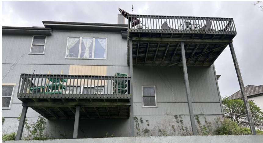
Figure 1 – Photo of existing decks.
