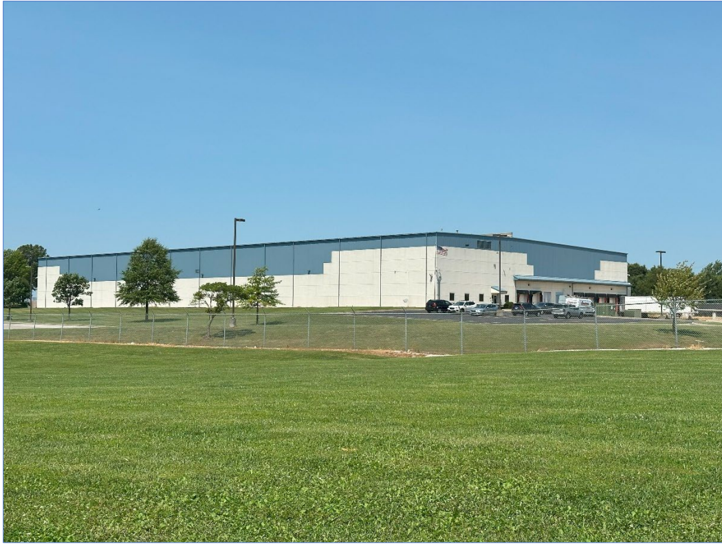
1 Pfizer Way – looking northwest from SE Bailey Rd – Zoetis Distribution Center
