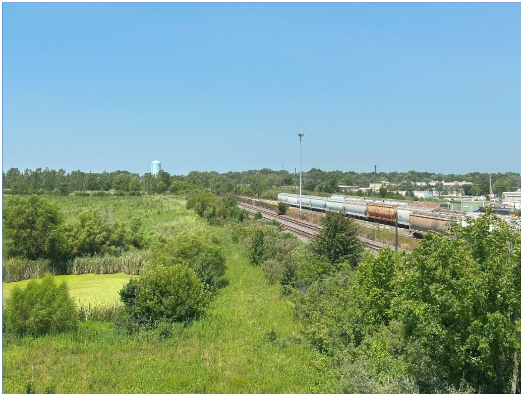
1 Pfizer Way – looking north along eastern property line – overgrown vegetation
