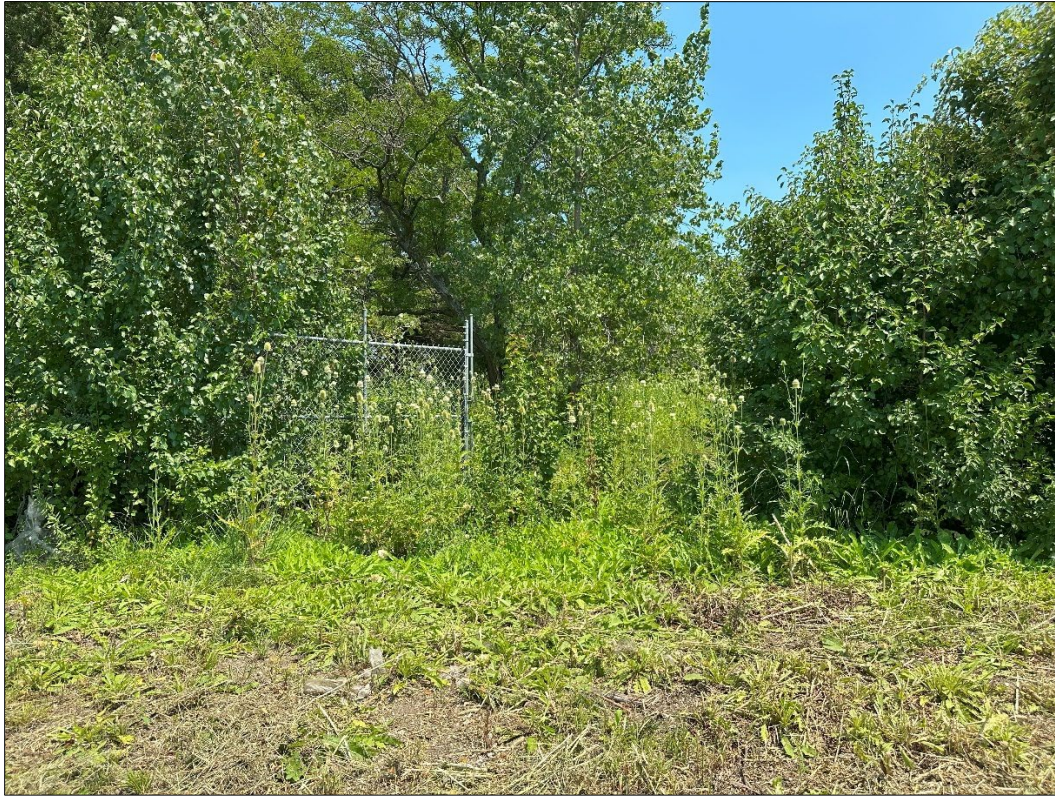
1 Pfizer Way – looking east – open gate; overgrown vegetation
