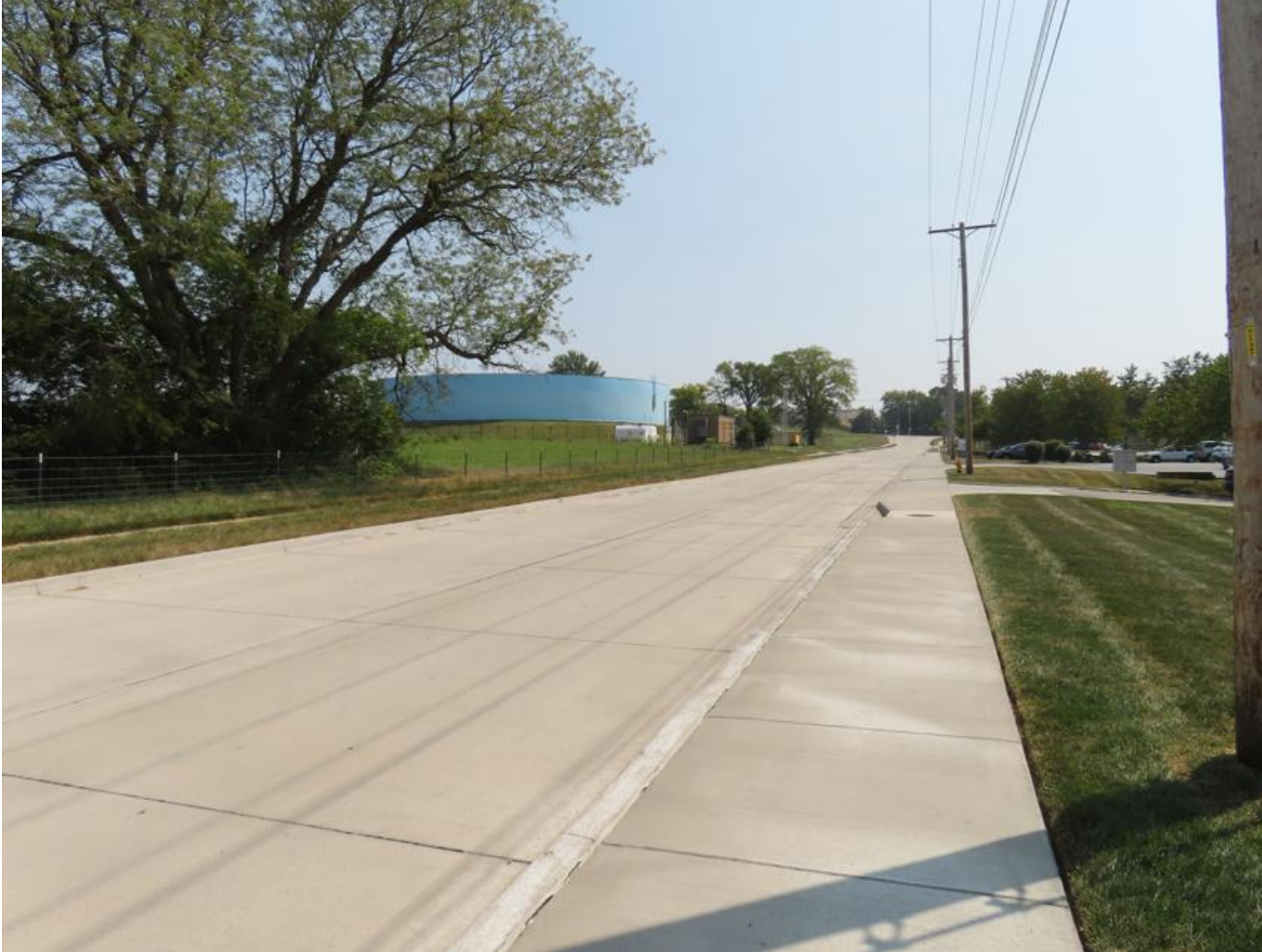
Looking from N.W. Main Street
