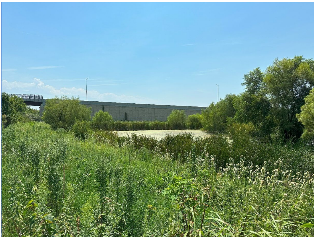
1 Pfizer Way – looking south – stagnant drainage pond; overgrown vegetation
