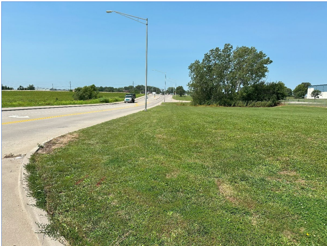
1 Pfizer Way – looking west – lack of pedestrian circulation (sidewalk) on north side of Bailey Rd
