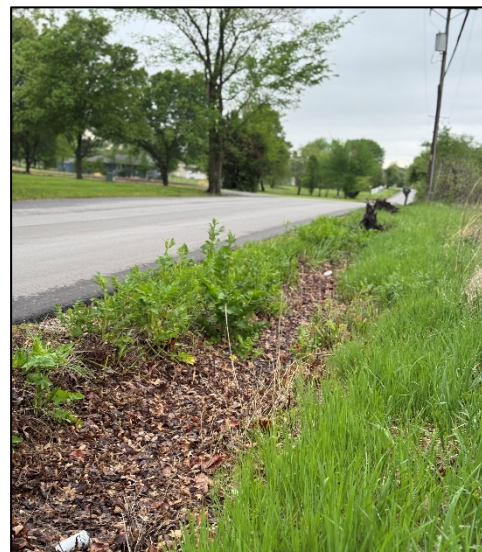
Prairie Rd & WB Site Drive Looking Right (N) – Left-Turn
