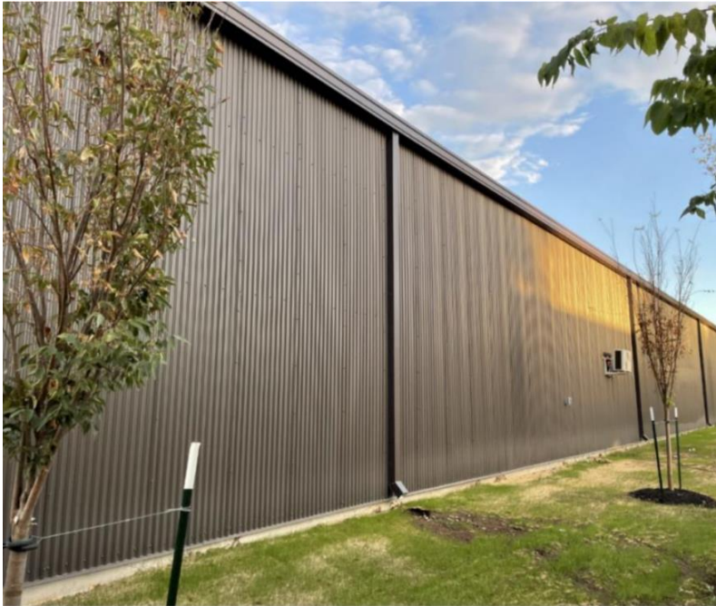
Rear elevation photo of identical project
