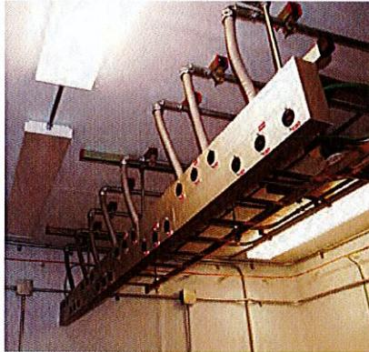
For convenient powering of the equipment, individual receptacles with dedicated power circuits are installed in a raceway system above the equipment racks.
