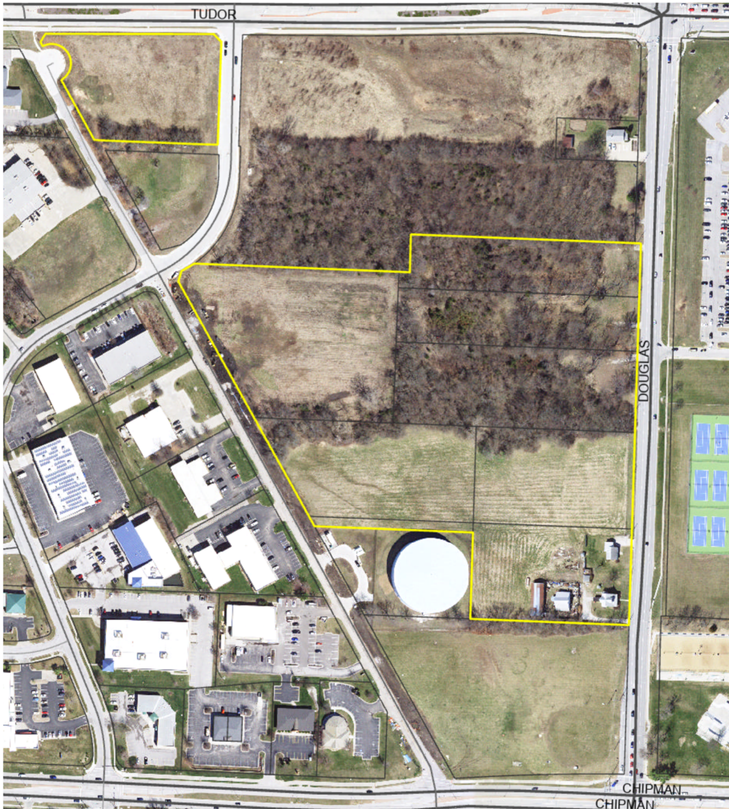
Figure 3 – Existing Conditions aerial
