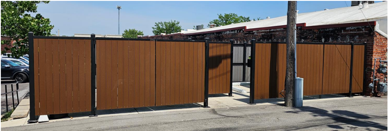
Figure 2 – Trash Enclosure at 216/218 SE Douglas St
