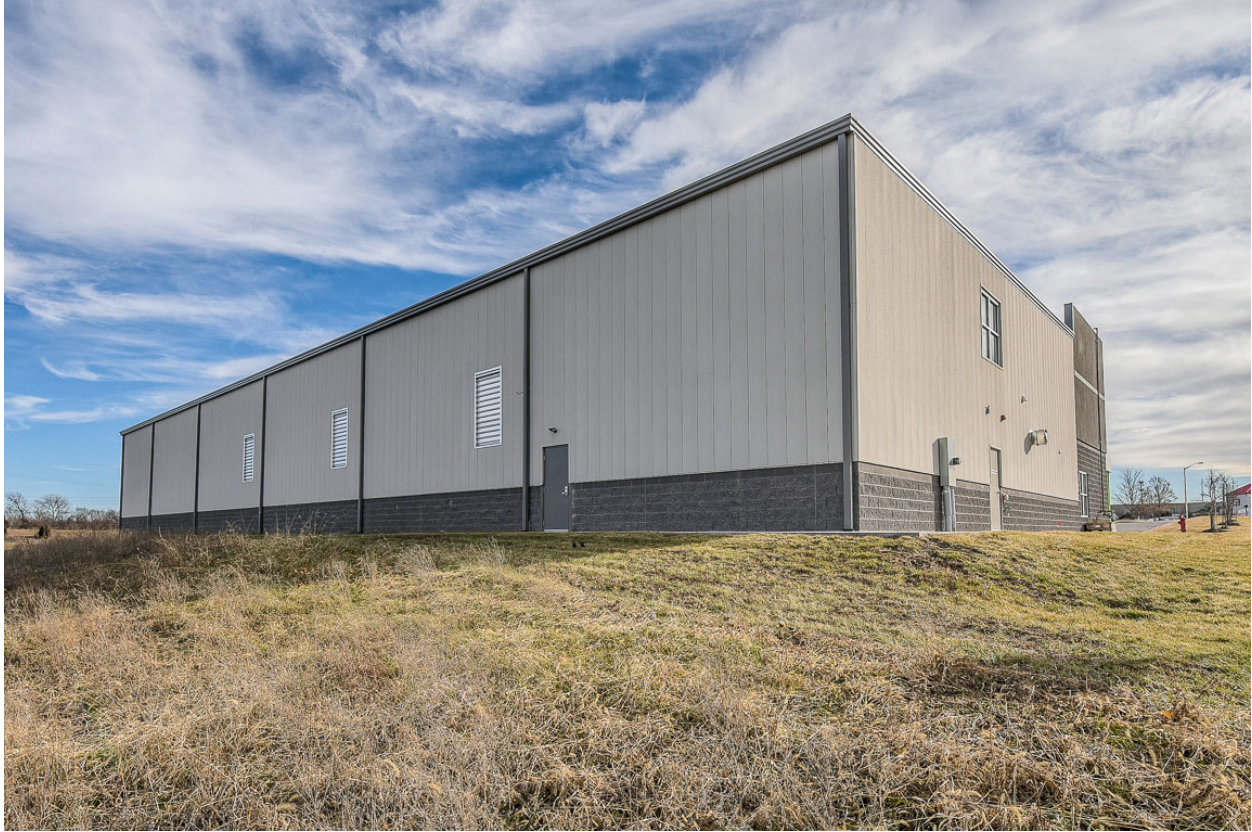
Textured Stucco finish flat metal wall panel, Pinnacle Gymnastics Facility, Shawnee, KS
