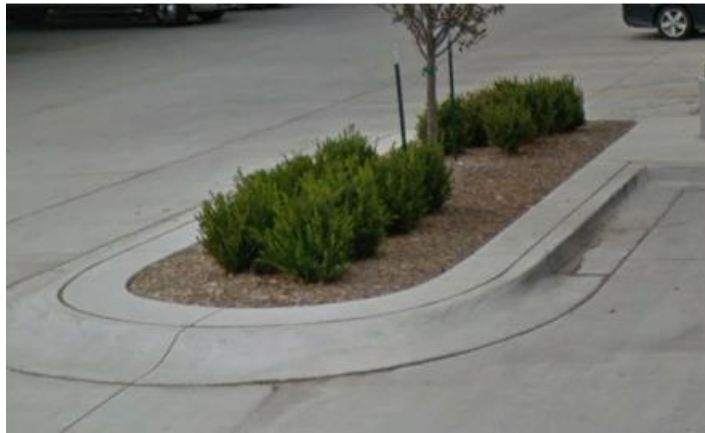
Figure 4 - Examples of proposed roll-over curbing for driveway radius (top) and landscape islands (bottom).
