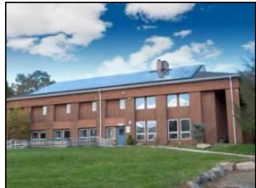
Commercial building with solar panels
