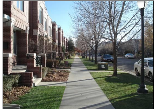
Ground-floor unit entrances
