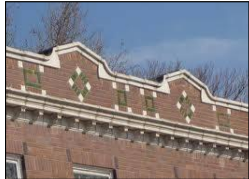
Parapet wall screening roof mounted equipment
