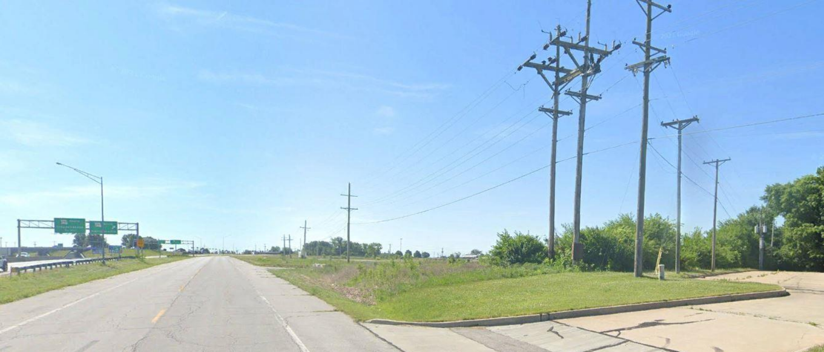
Looking East at Northeast Corner
