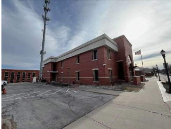
Photo #1 Facing E: Overview of site from W corner
