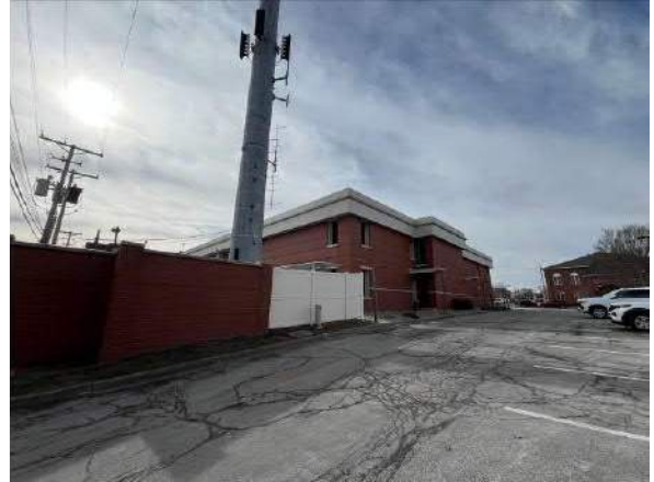
Photo #2 Facing S: Overview of site from N corner
