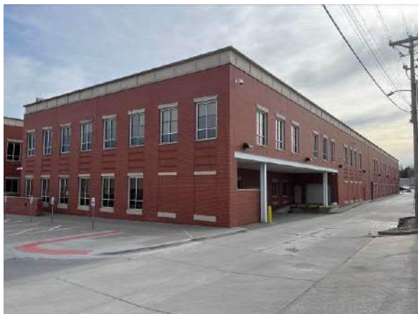
Photo #23 View of E-adjacent City Hall
