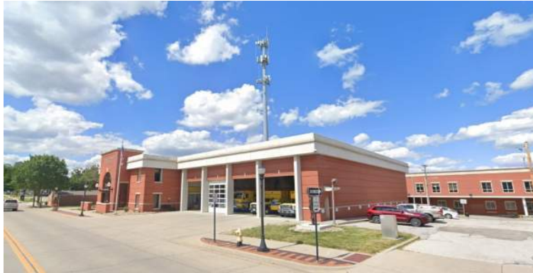
Original building was constructed in 1974, Building has undergone renovations throughout its 50 year lifespan. A brick façade was added to the structure in 2005 and some minor interior renovation work was completed that same year.
