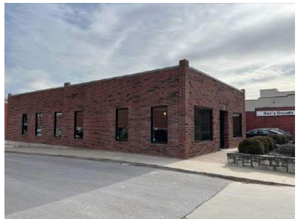
Photo #24 View of SE-adjacent vacant commercial building
