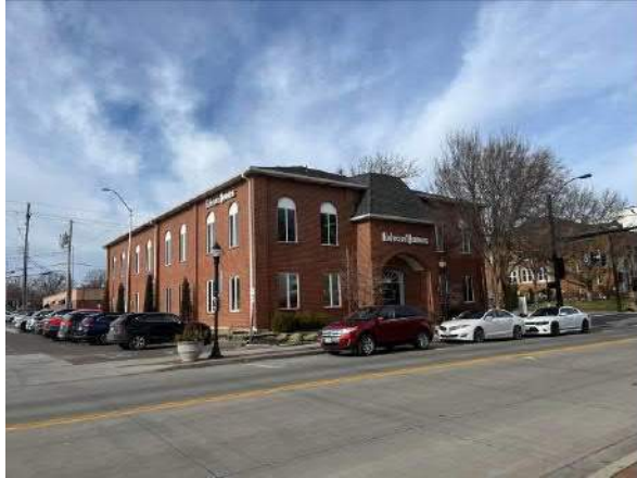
Photo #19 View of WSW-adjacent Edward Jones
