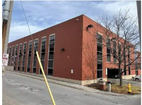
Photo #22 View of NE-adjacent parking garage
