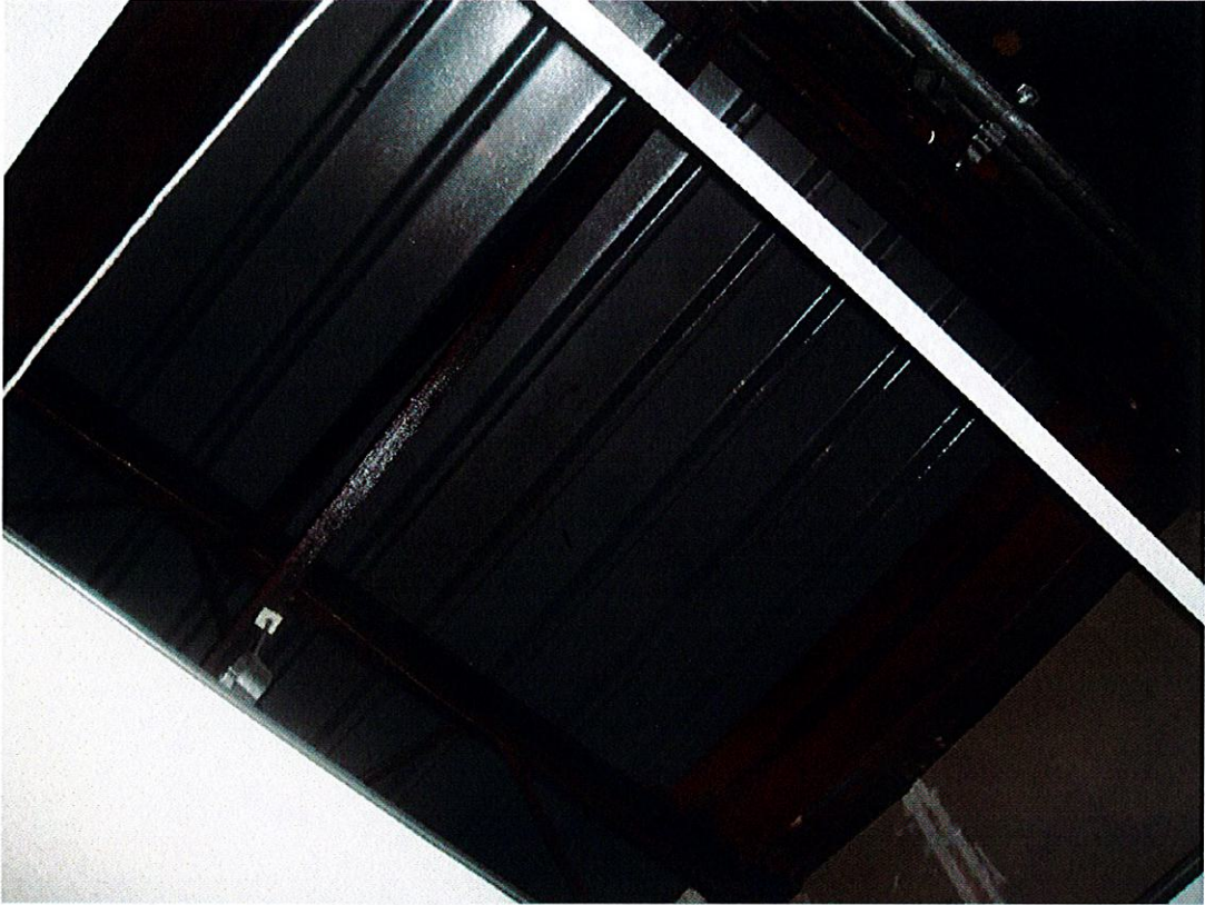
Photo 32 – Roof structure condensation.
