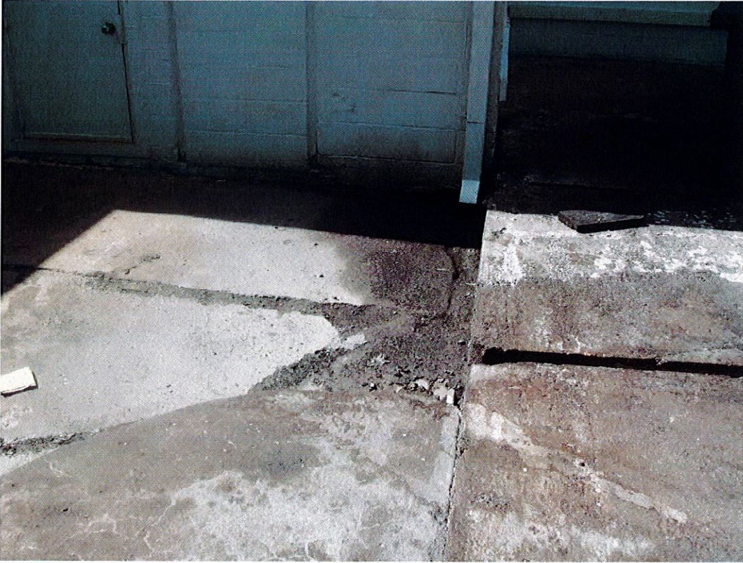
Photo 20 – Inadequate drainage.
