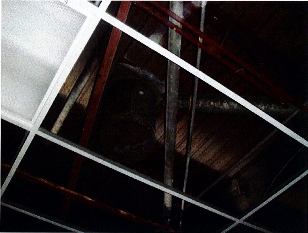
Photo 28 – Roof structure deterioration.
