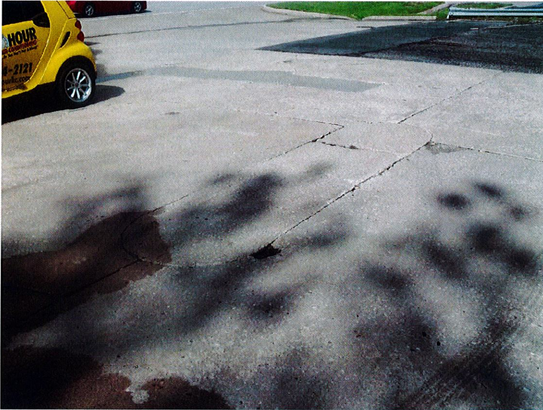
Photo 40 – Former gas pump location.
