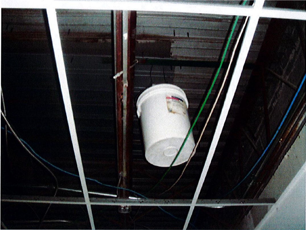
Photo 27 – Roof structure deterioration.
