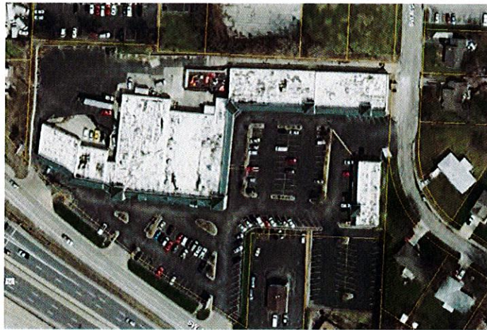
Figure 9 - Before Picture Roof Condition: Year 2010.
