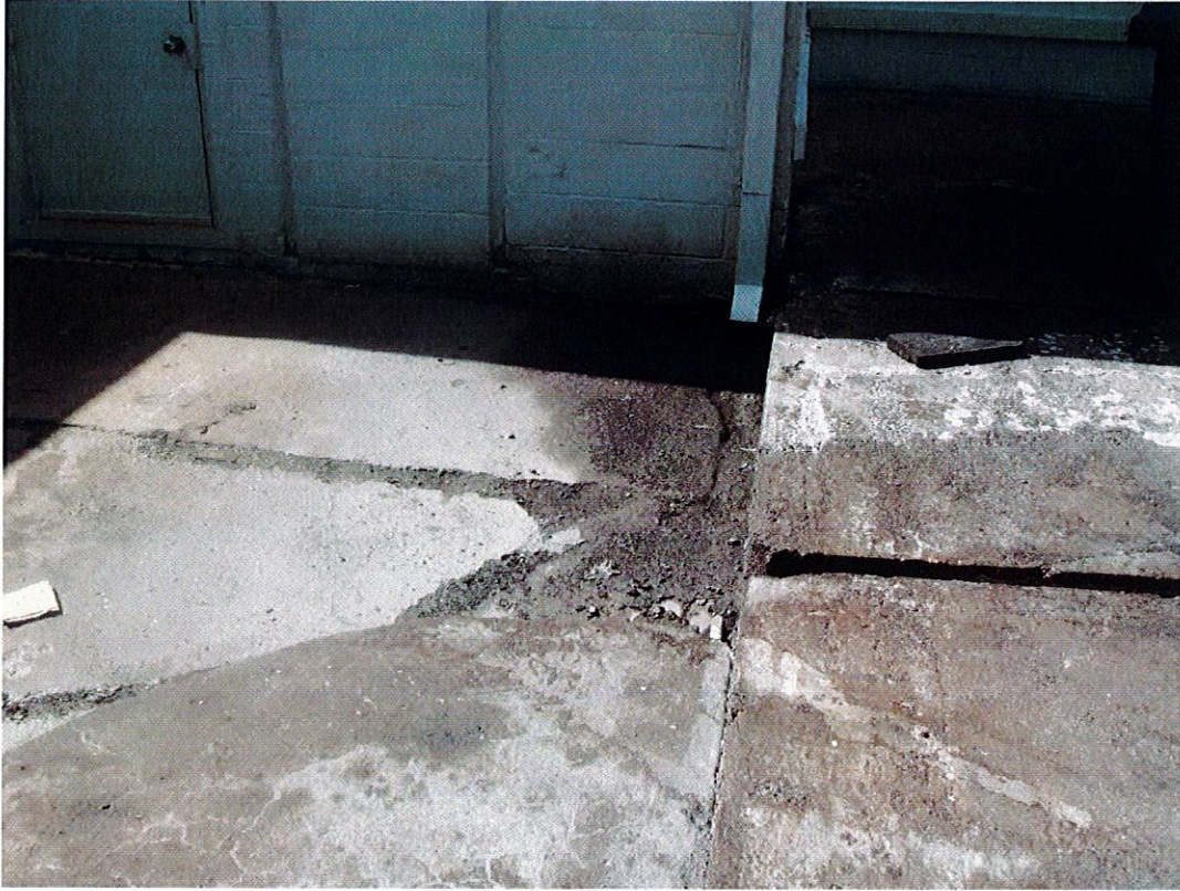
Photo 20 – Inadequate drainage.
