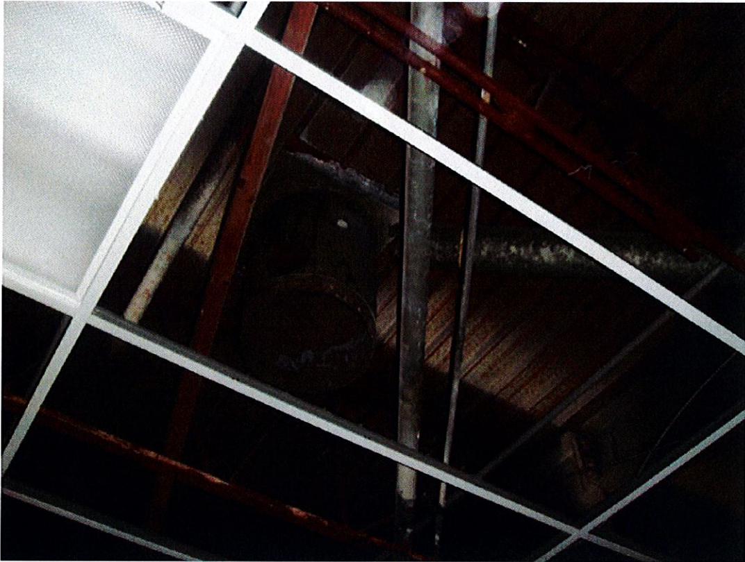
Photo 28 – Roof structure deterioration.
