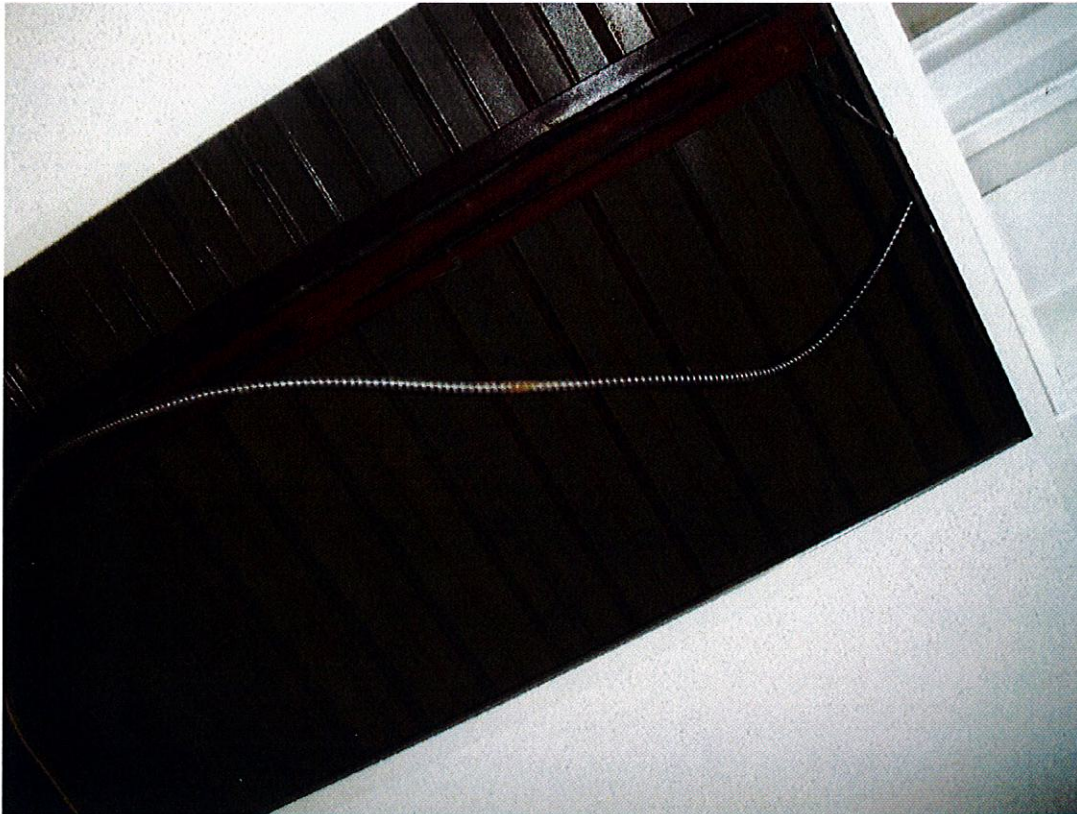
Photo 30 – Roof structure condensation.
