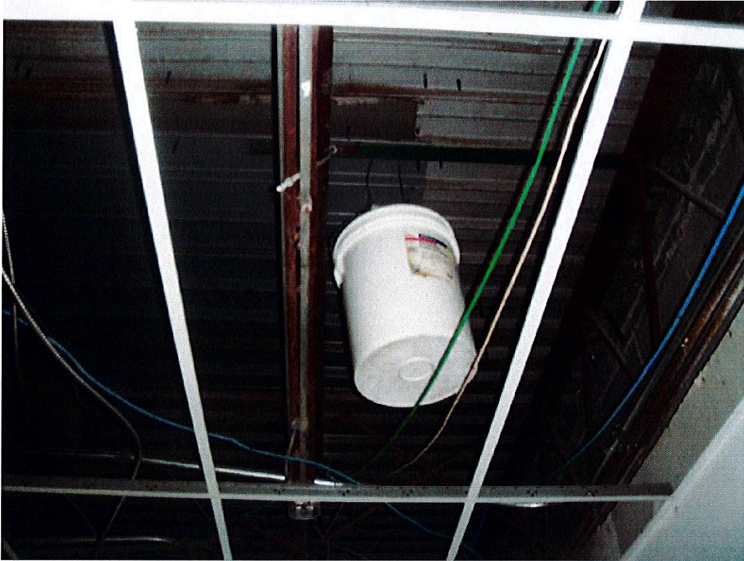
Photo 27 – Roof structure deterioration.
