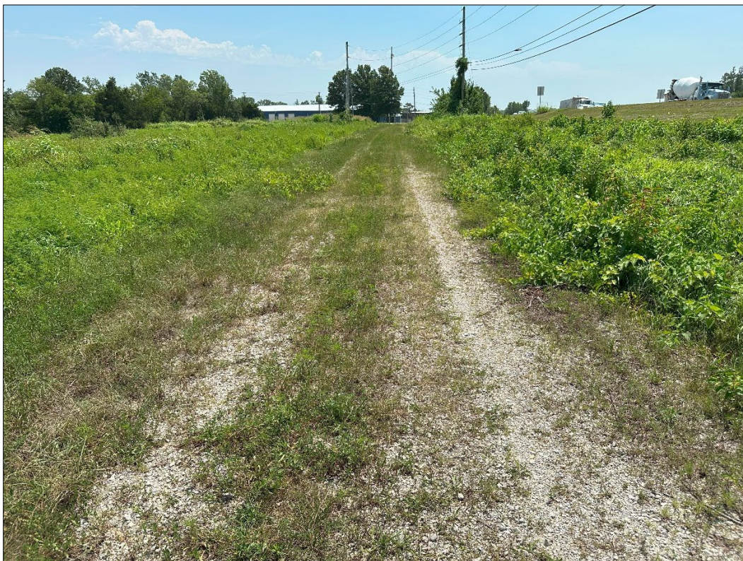
SEC M-291 and SE Bailey Rd – looking south – deterioration of access road
