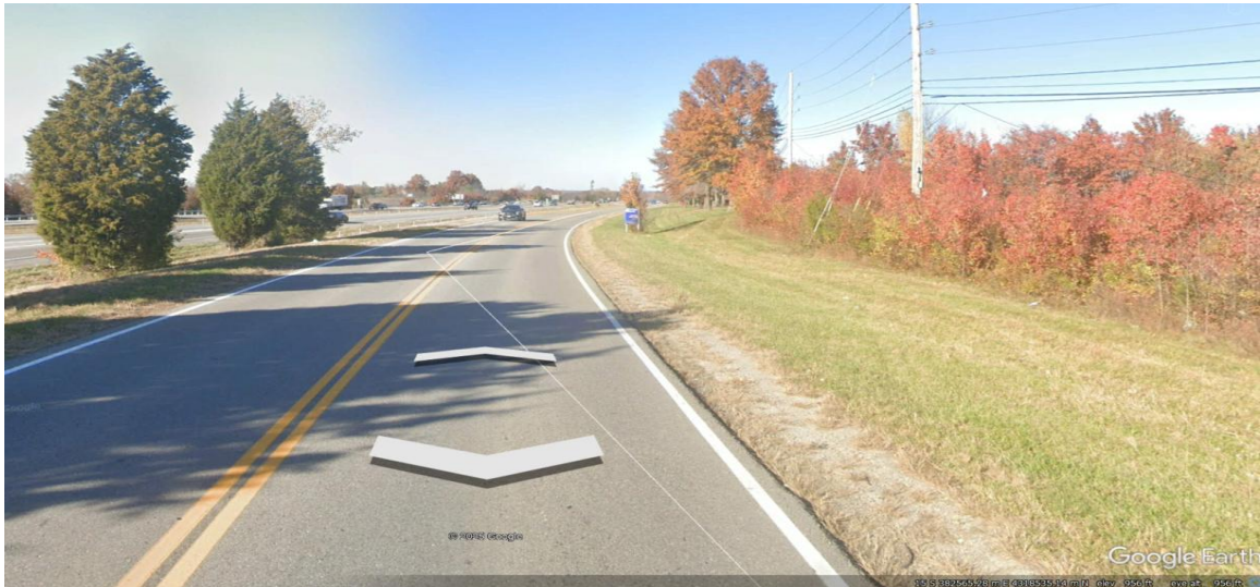
Proposed North Driveway Looking North. Obtained from Google Earth Street View.
