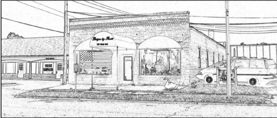
One-story Tapestry Brick commercial building at 110 SW 3rd Street. This building features an intact storefront and corbelled brick cornice.
