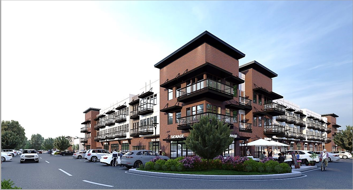
CORNER – 150 Highway & Pryor Road
