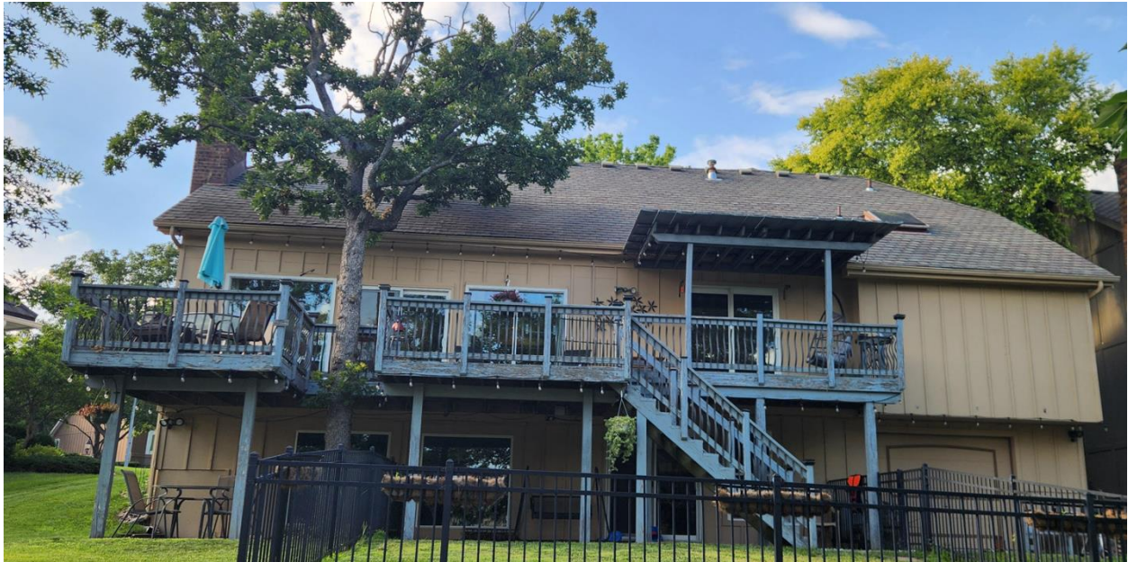
Figure 1 – Photo of existing deck.
