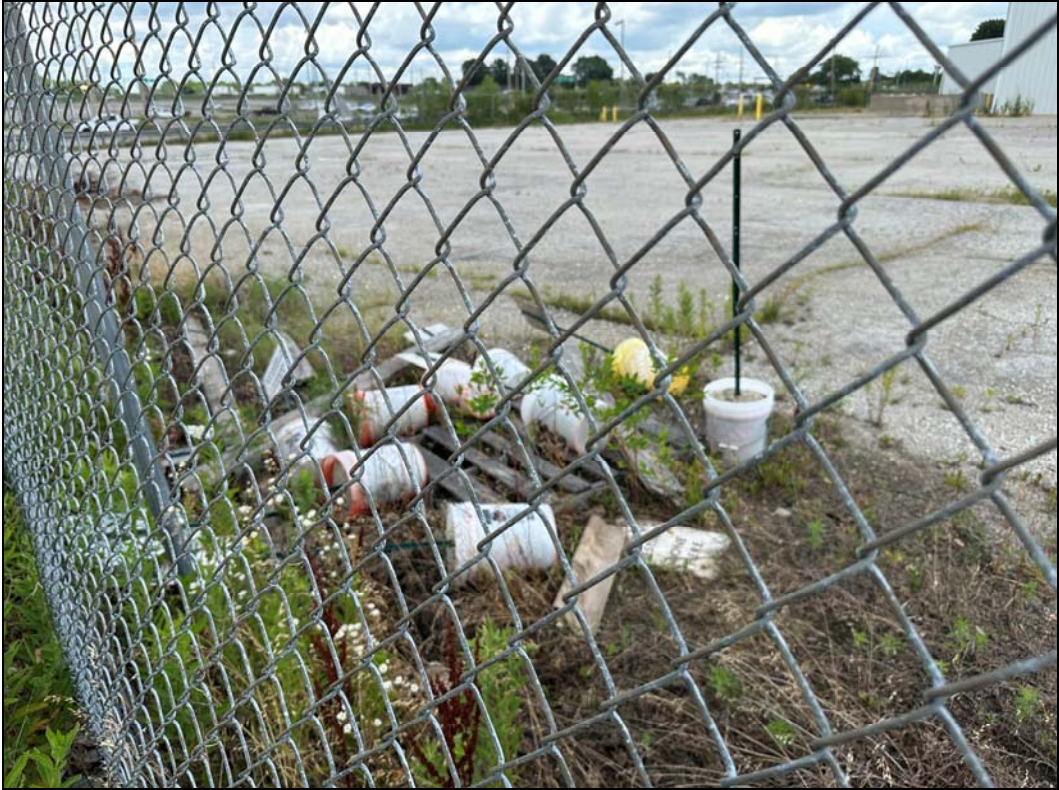
1204 SW Jefferson St – trash/debris; deterioration of pavement
