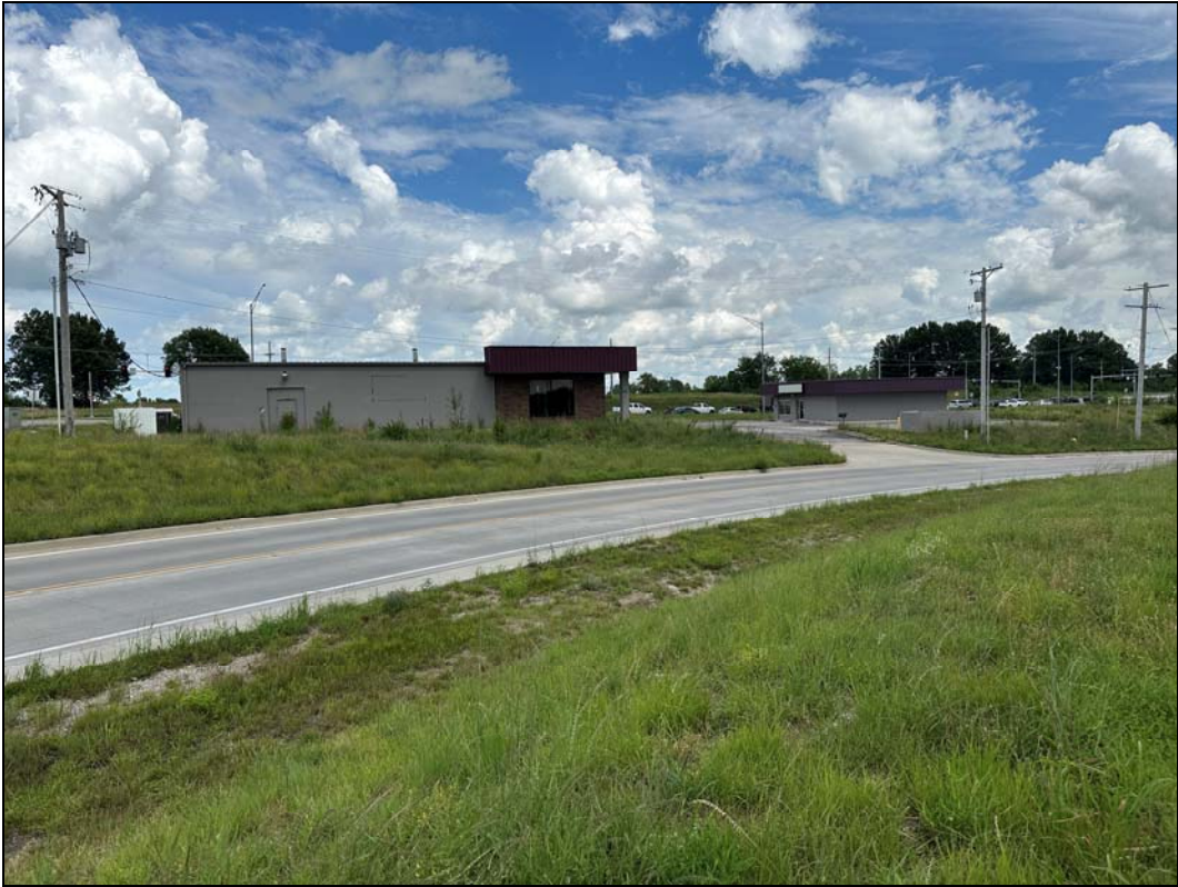
1025-1031 SW Jefferson St – overgrown vegetation; lack of pedestrian circulation
