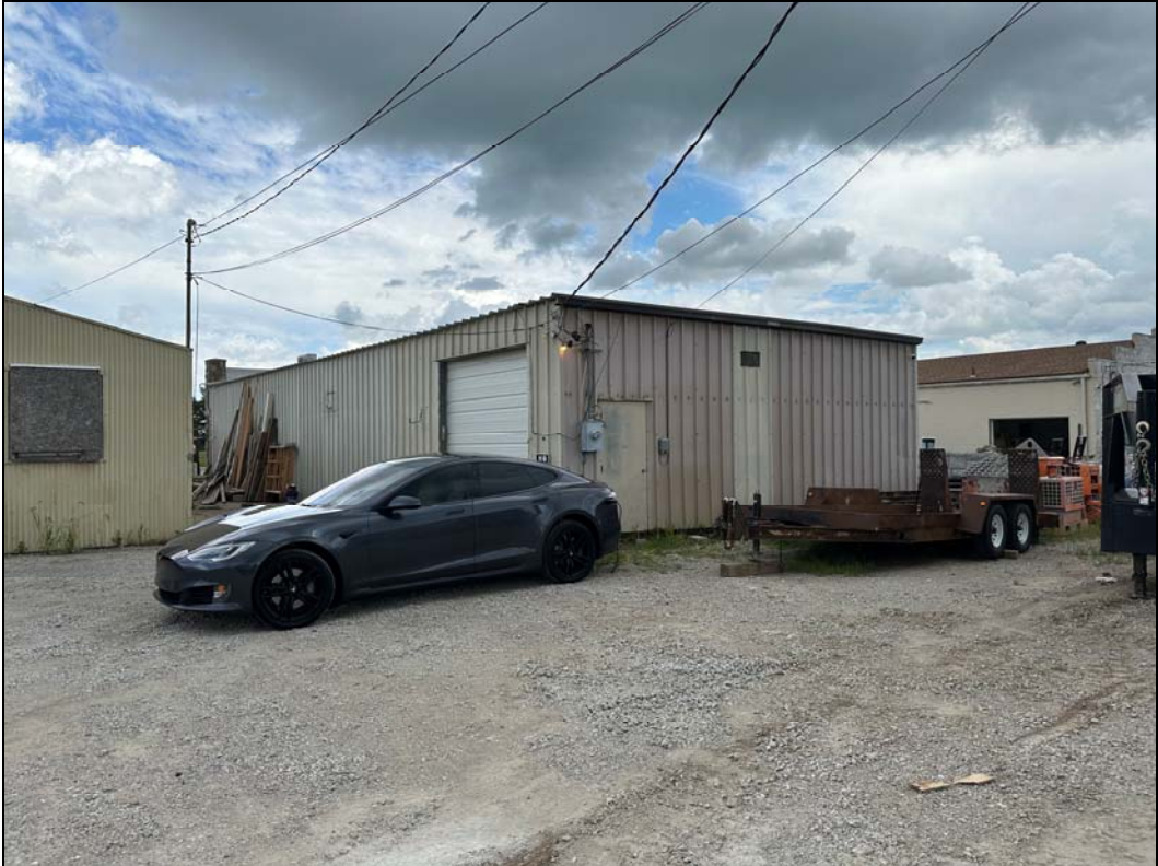
1302 SW Market St – failure of finishes; deterioration of pavement
