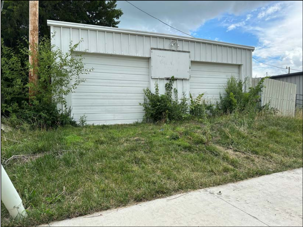
1212 SW Market St – overgrown vegetation; trash/debris
