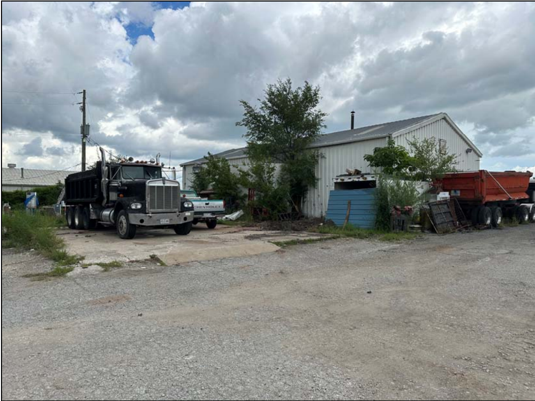
1301 SW Jefferson St and 1212 SW Market St – deterioration of pavement
