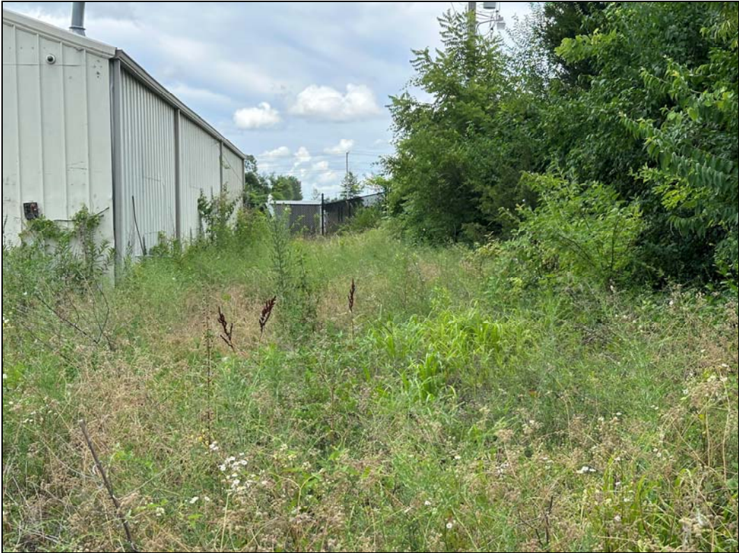
1210 SW Market St – overgrown vegetation
