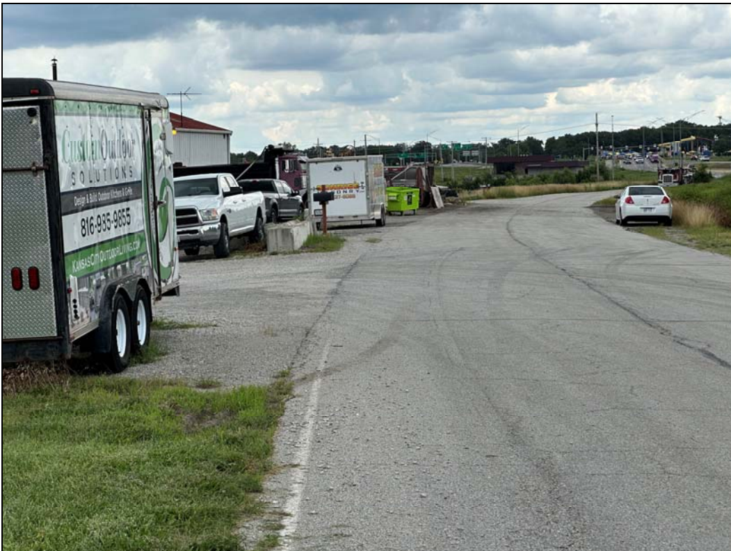
1304 SW Market St – lack of standard curbs and driveways (too wide)
