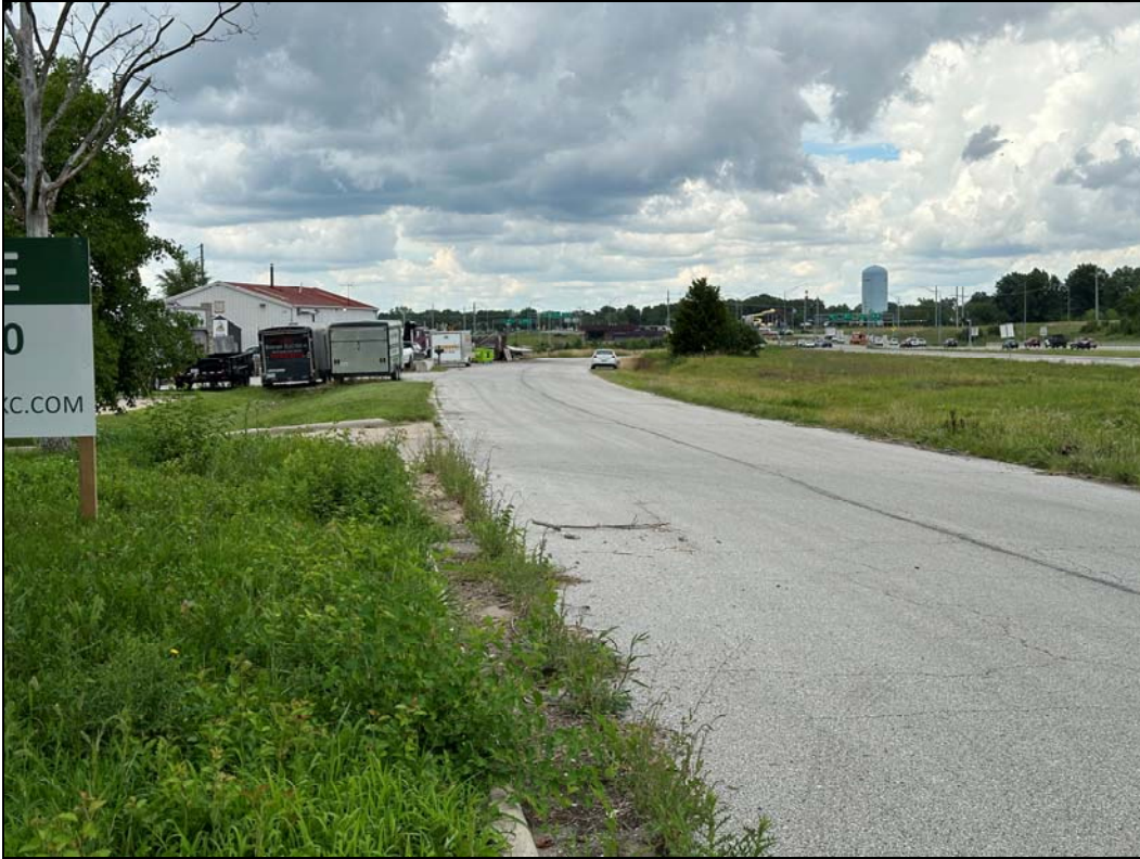
1306 SW Market St – overgrown vegetation; lack of standard curbs and driveways
