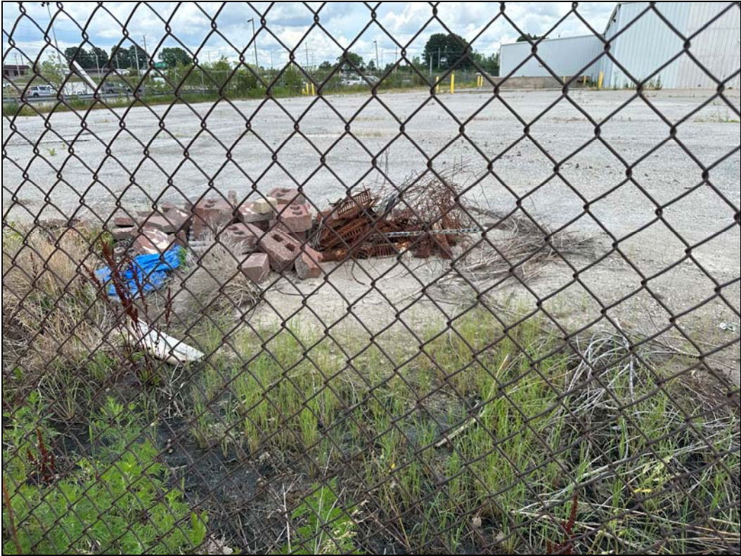
1204 SW Jefferson St – trash/debris; deterioration of pavement
