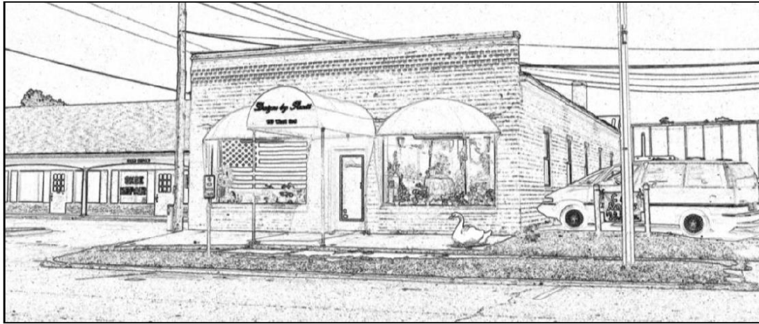
One-story Tapestry Brick commercial building at 110 SW 3rd Street. This building features an intact storefront and corbelled brick cornice.
