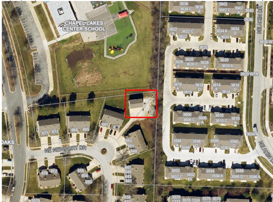
Figure 1: Aerial View of the Chapel Oaks Maintenance Storage facility (subject property outlined in red)
