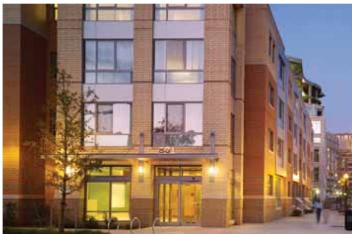
The Jordan is a complex of 90 affordable apartments in Arlington, Va., acquired through land a swap with JBG Companies. Amenities include a community center, water play area for children, a library and a public transit subsidy for residents. (Photo courtesy of Harkins Builders)
