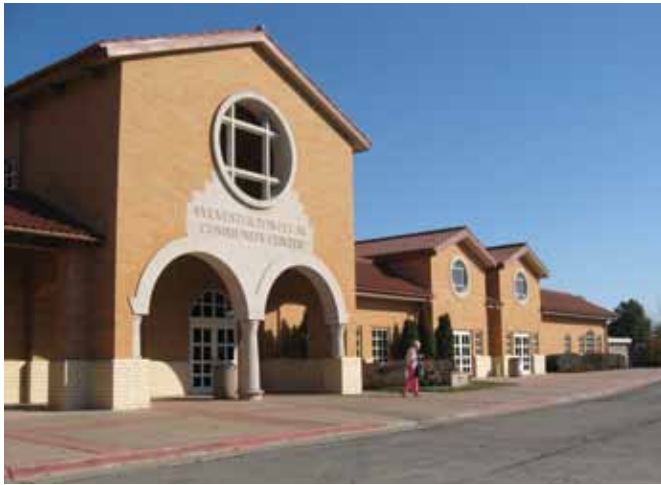
Sylvester Powell, Jr., Community Center in Mission, Kan., offers physical fitness facilities, classes and meeting spaces for community forums and other events.
