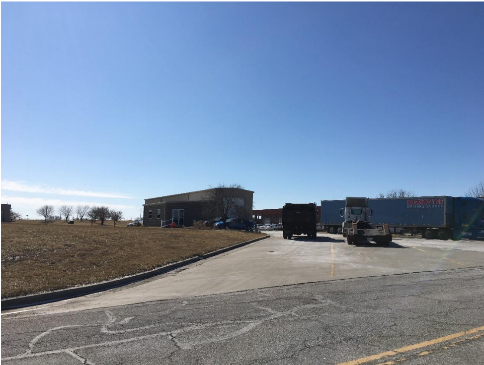
MODOT Service facility south of Town Center Drive
