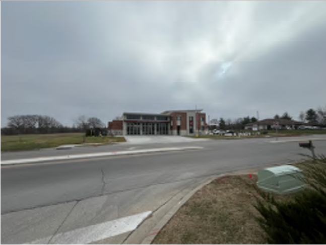
25. Fire department on NE Lakewood Way
