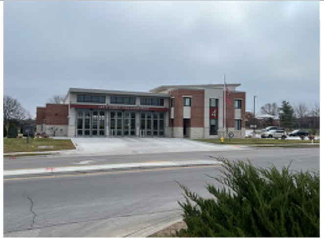
26. Fire department on NE Lakewood Way
