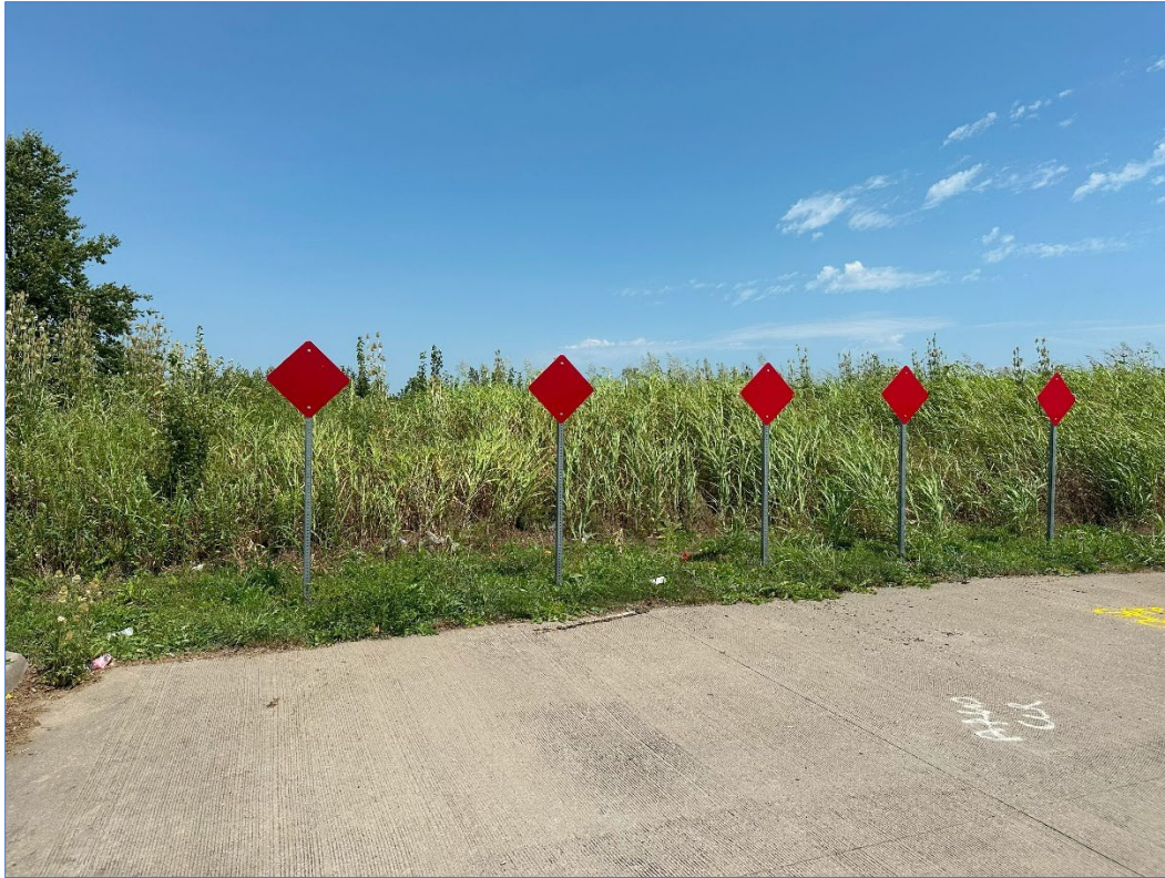
1 Pfizer Way – looking north from SE Bailey Rd – overgrown vegetation
