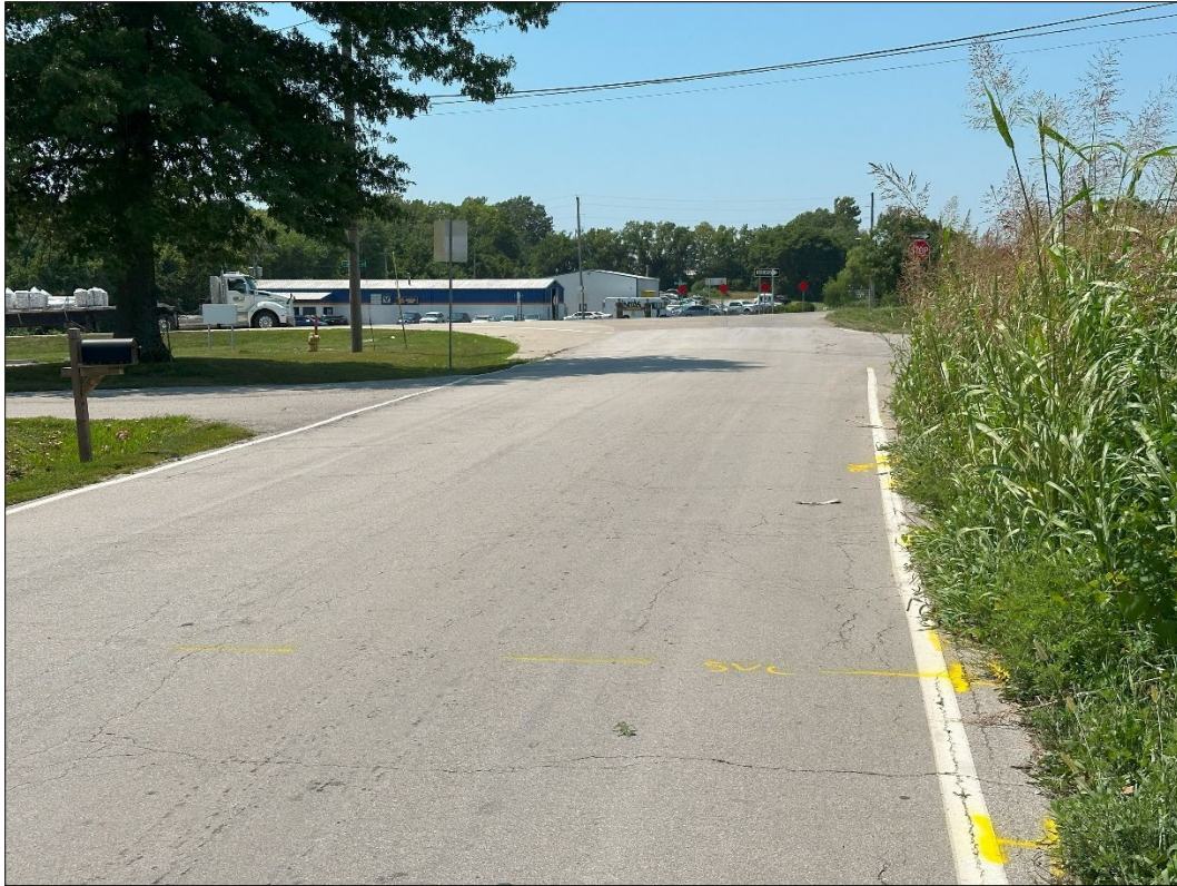
4 SE 16 th St – looking west – overgrown vegetation encroaching on 16 th St
