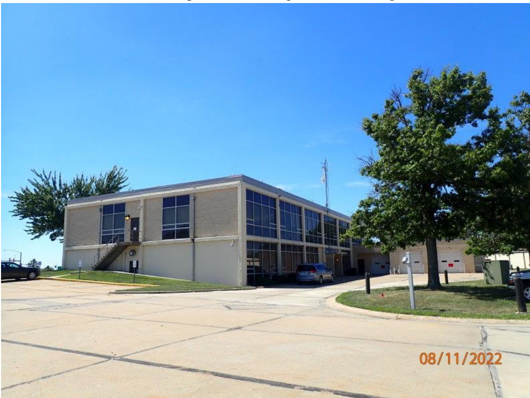
View of the side and rear of the headquarters building. Camera facing southwest.
