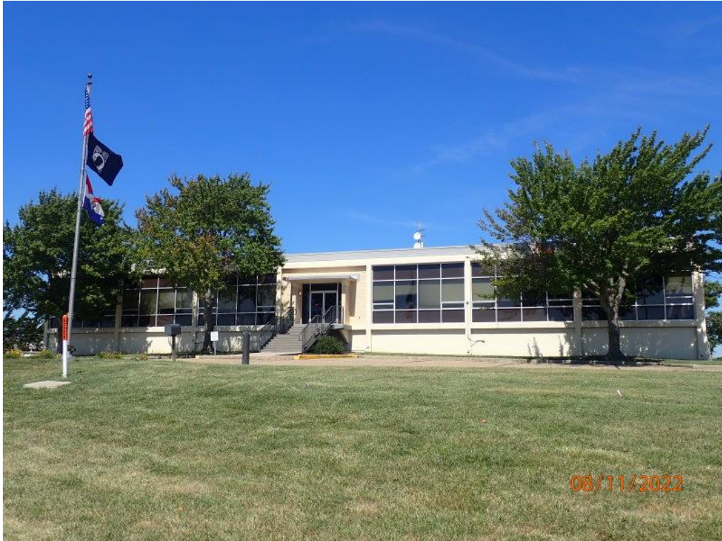
View of the front entrance to the headquarters building. Camera facing northwest.
