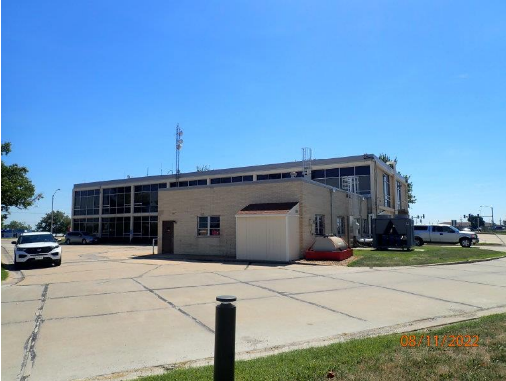
View of the rear of the headquarters building. Camera facing southeast.
