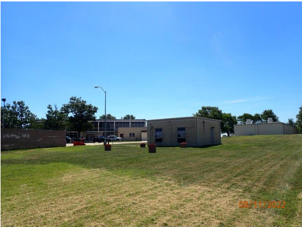
View from the northern boundary of the parcel, showing all three buildings with the communication building in the foreground. Camera facing south.
