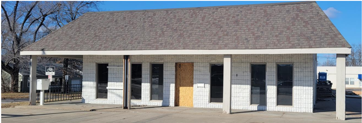
Figure 2 – Existing south façade of the subject building
