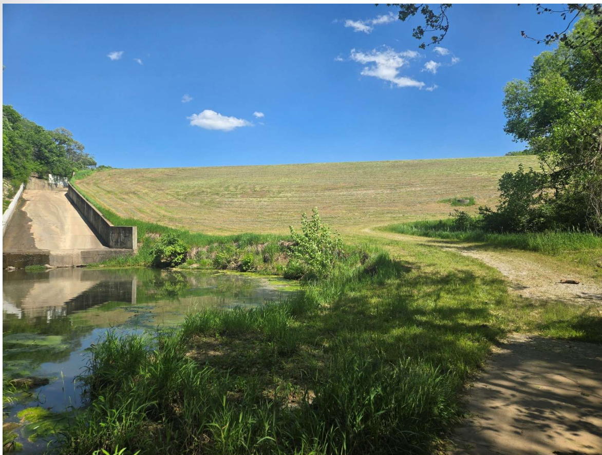
Left: Unity Lake #2, Regional Detention Basin in Unity Village, Jackson County, MO. Height: 52 feet. Length: 450 feet. Storage: 618 ac-ft.
