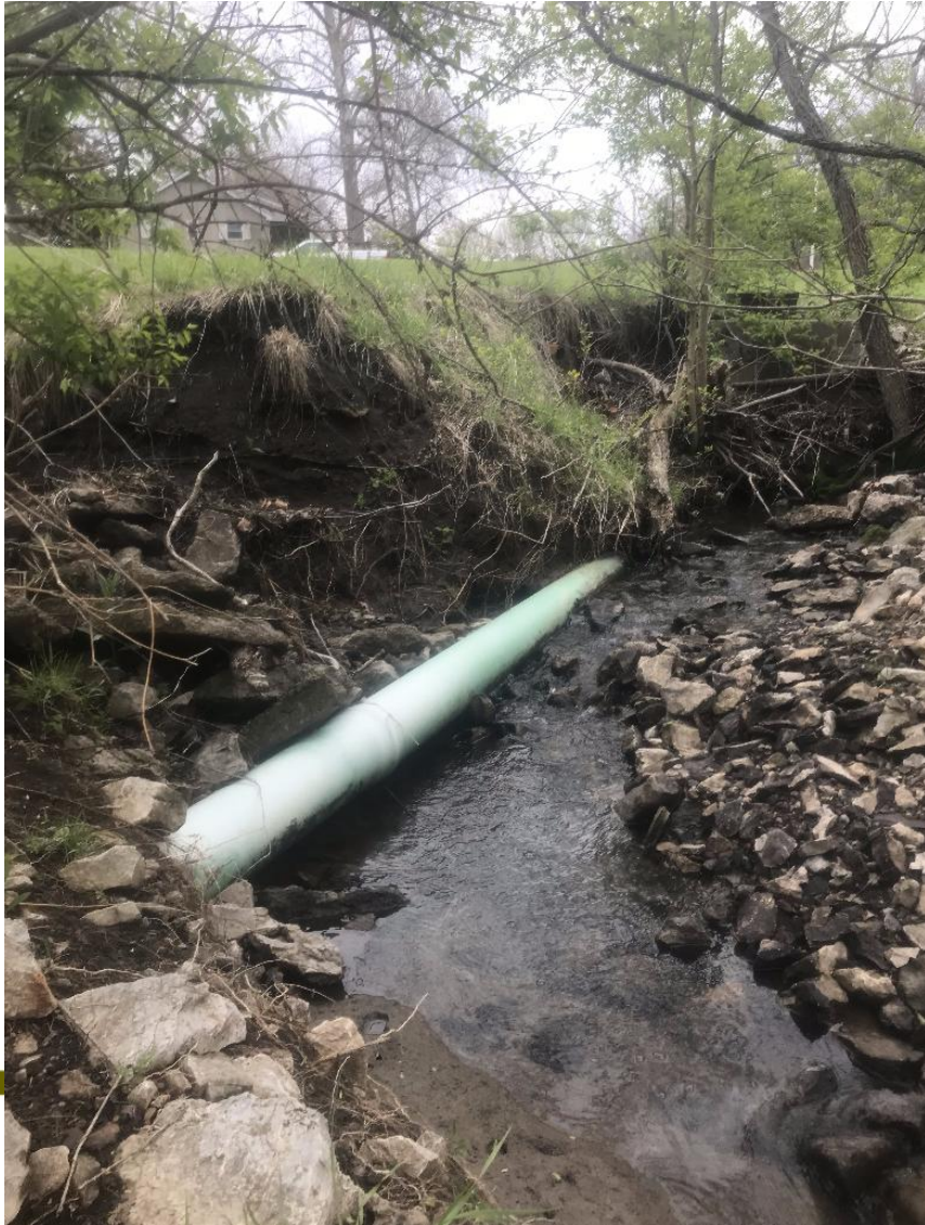
Exposed Sewer Main
