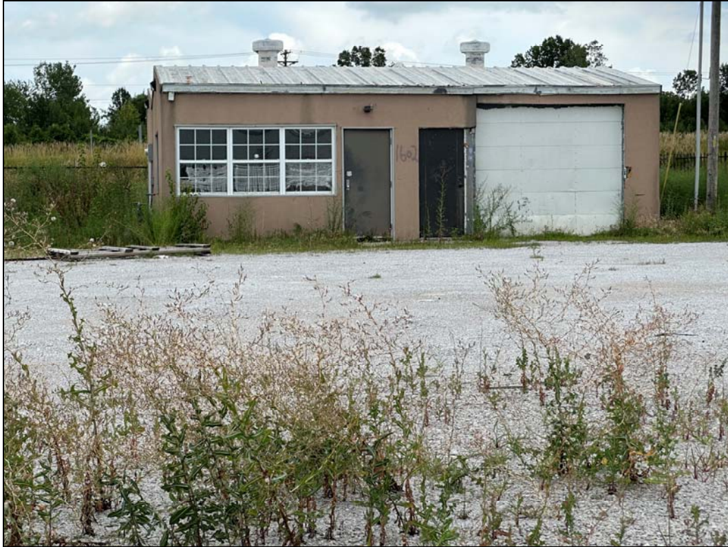
1206 SW Market St – deterioration of roof, fascia, gutter and downspouts, doors, and failure of finishes
