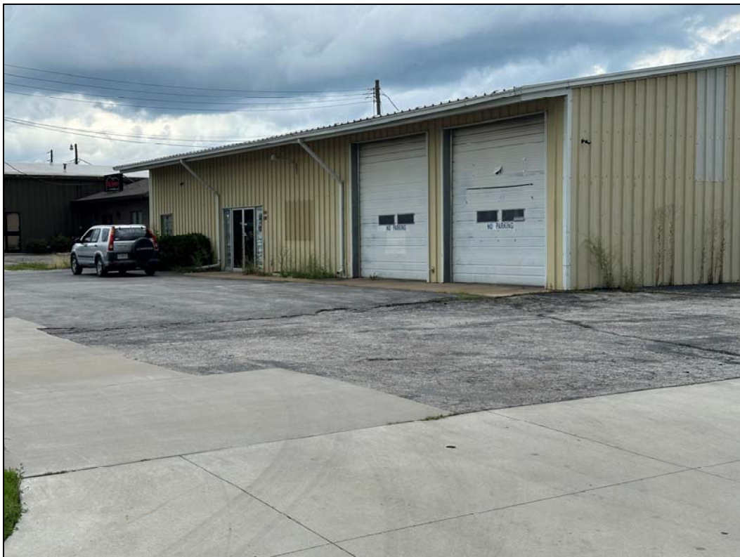
1313 SW Jefferson St – deterioration of doors; failure of finishes; deterioration of pavement
