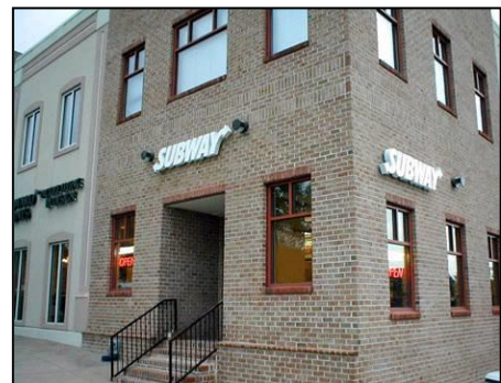
Fig. 6.480.B-28: Franchise design consistent with surrounding structures
