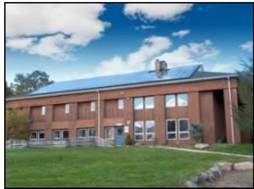
Fig.6.480.B-34: Commercial building with solar panels
