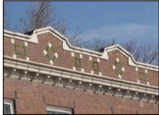
Fig. 6.480.B-5: Parapet wall screening roof mounted equipment
