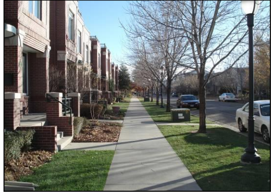
Fig.6.480.B-15: Ground-floor unit entrances
