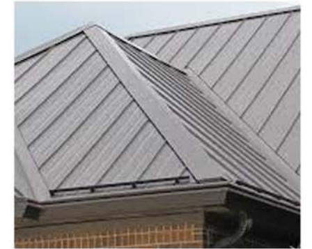
Standing Seam Metal Roofing
