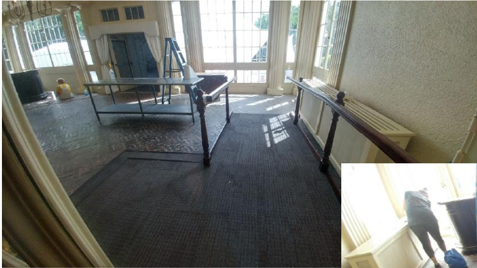
New platform and ramp, looking from the Hall into the Loggia
