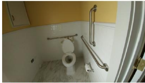
Renovated Bathroom, 1 st floor
