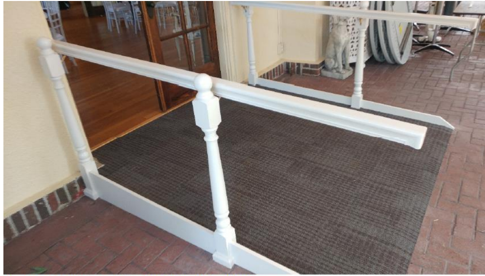
New ramp in west porch leading to the Living Room
