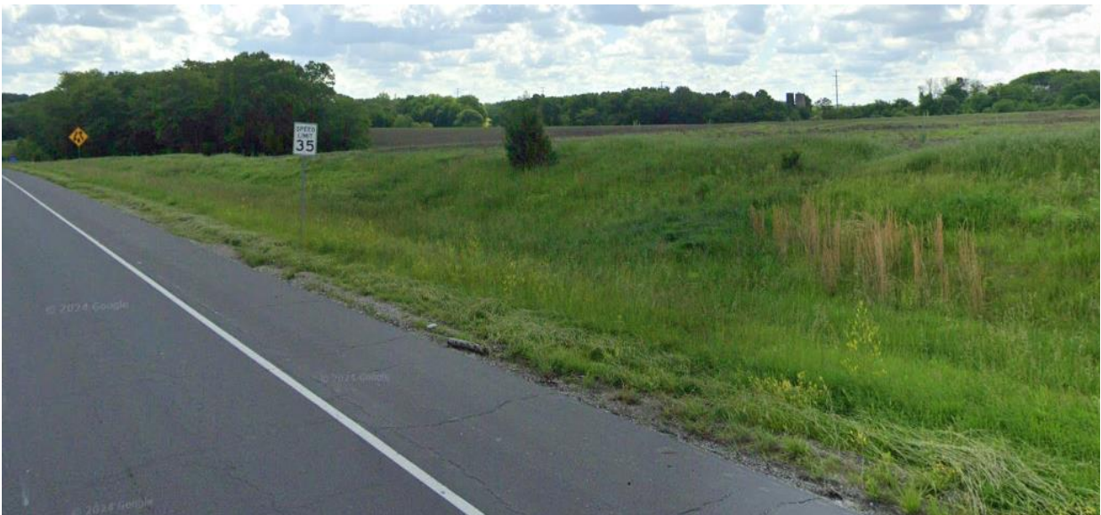
Unsecured and Unlit Property Boundary along NE Strother Road
