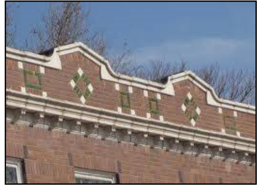
Fig. 6.480.B-5: Parapet wall screening roof mounted equipment
