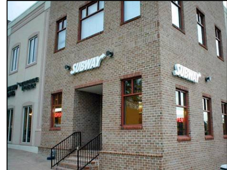
Fig. 6.480.B-28: Franchise design consistent with surrounding structures
