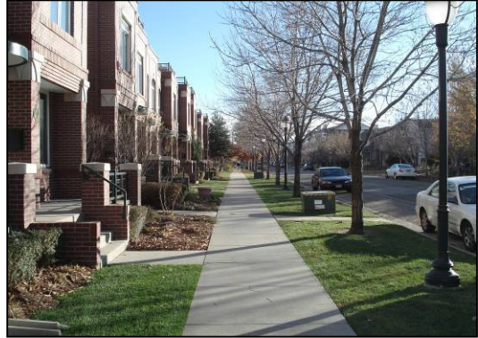
Fig.6.480.B-15: Ground-floor unit entrances
