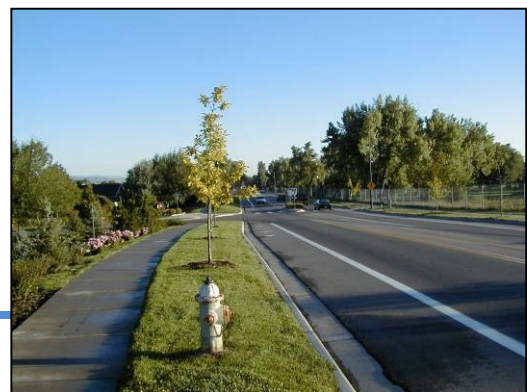
Fig. 6.480.B-1: Sidewalks on both sides of street
