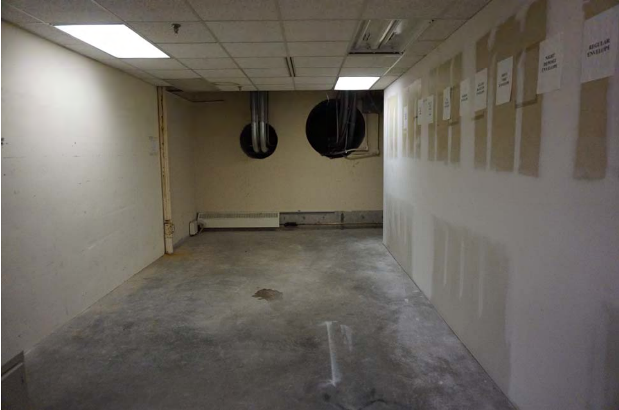
Representative interior view of unfinished space
