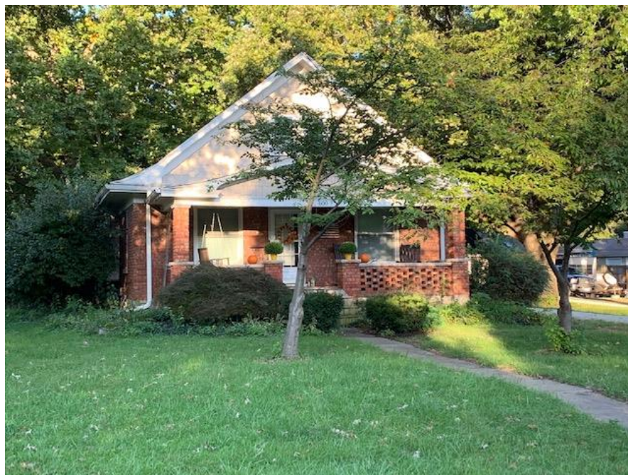
Existing Bungalow with Front Porch
